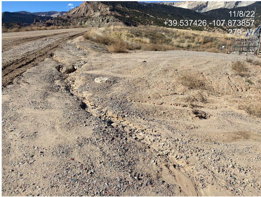
Photo 6. Photo shows rill erosion occurring on the road and pad surface.
