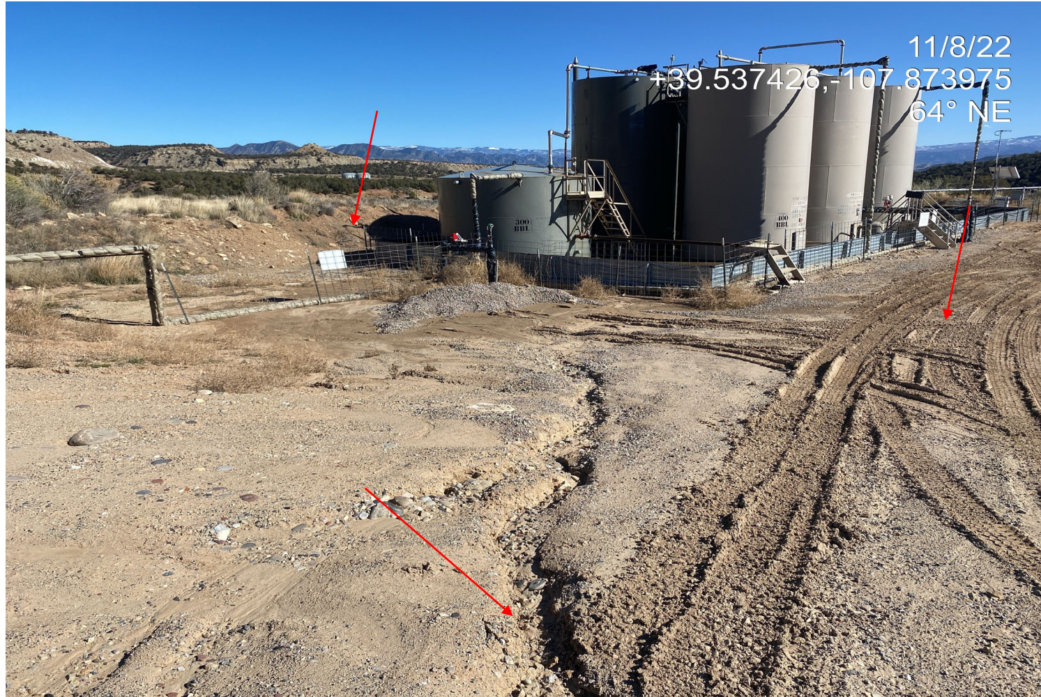
Photo 8. Photo shows lack of stabilization/compaction (ruts), rill erosion occurring in the road and pad surface and unstabilized cut slopes.
