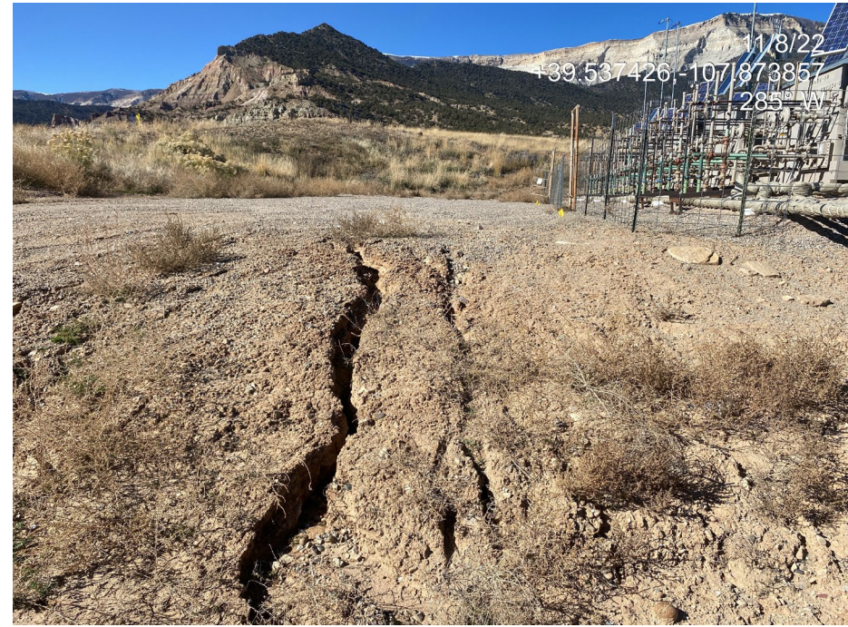
Photo 7. Photo shows rill erosion in the slopes adjacent to the separators.
