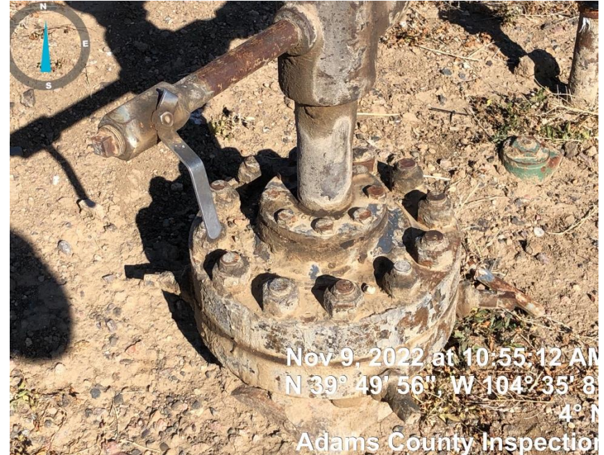
Photo#4 Leaking Gas below Master Valve
