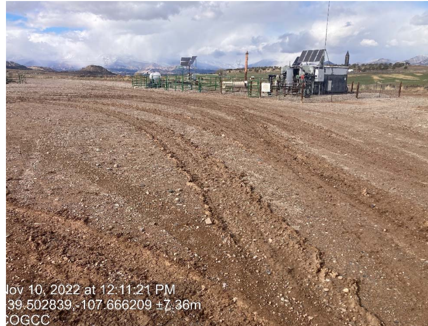
Lack of stabilization/ compaction
