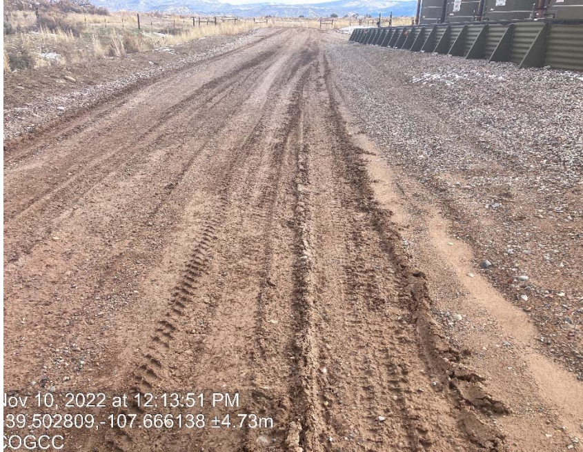
Lack of stabilization/ compaction
