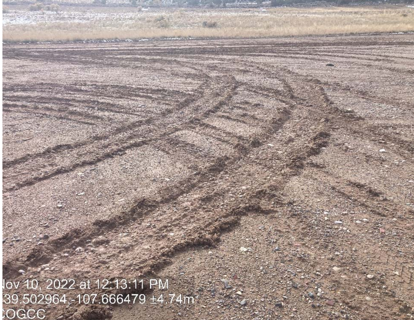
Lack of stabilization/ compaction
