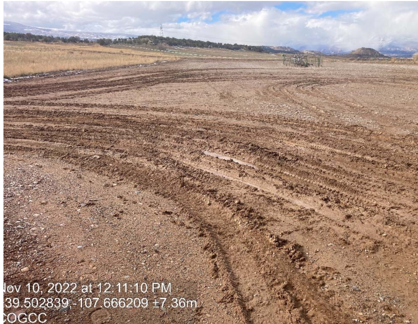
Lack of stabilization/ compaction
