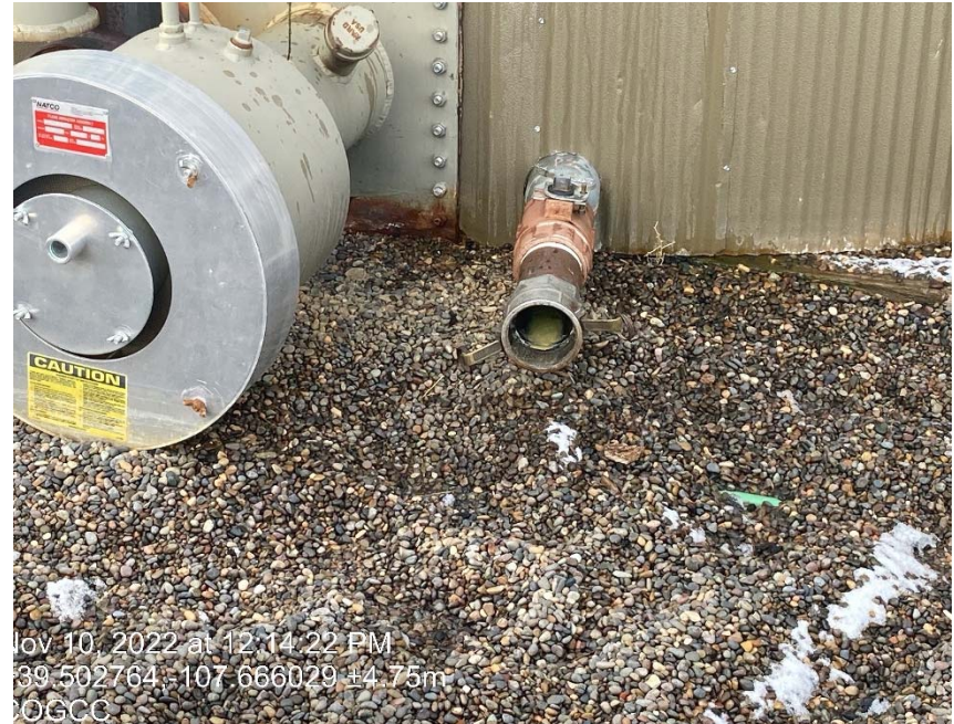
Missing plug/cap
