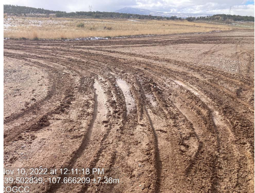
Lack of stabilization/ compaction
