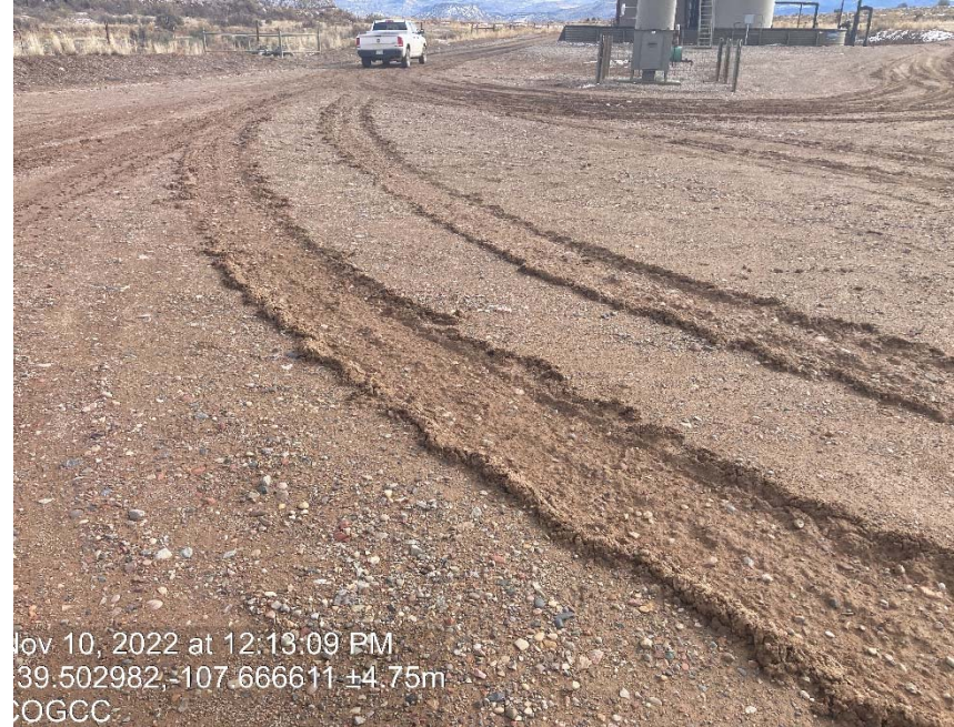
Lack of stabilization/ compaction
