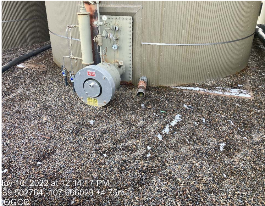
Missing plug/cap
