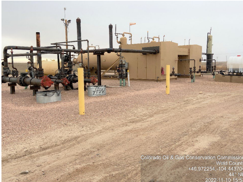
Photo #5 Fox Creek /33 NWNW 2: Wellsites SW Pad Separators, Gas Lift manifold
