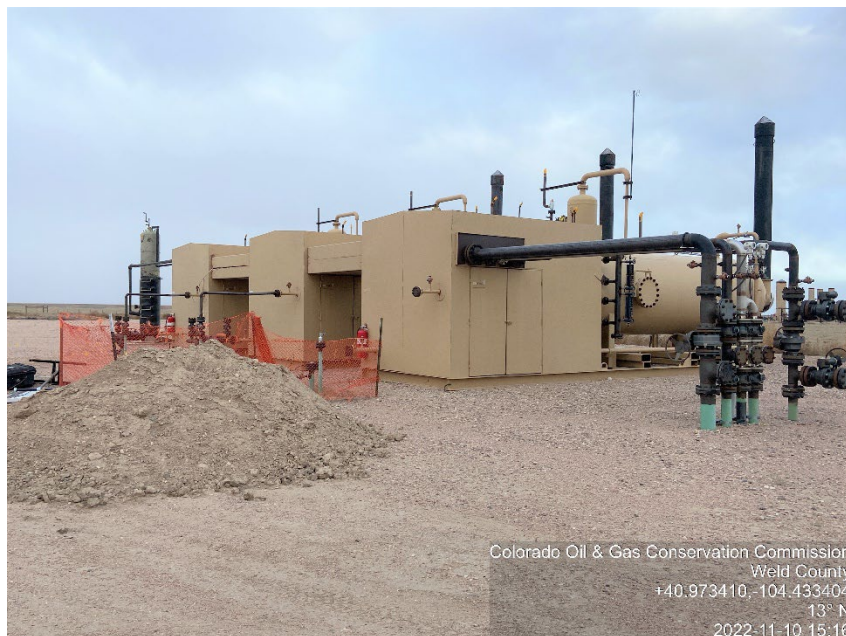
Photo #5 Fox Creek /28 SWSE 2: Wellsites W Pad Separators, Gas Lift manifold
