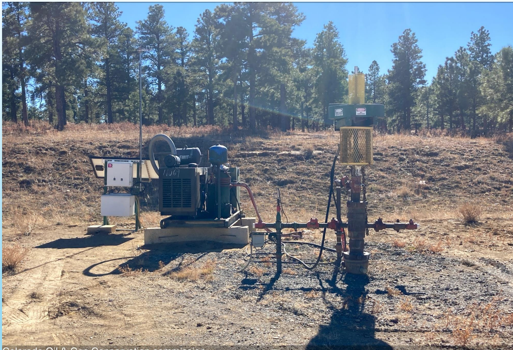
PHOTO 3: WELLHEAD AND EQUIPMENT
