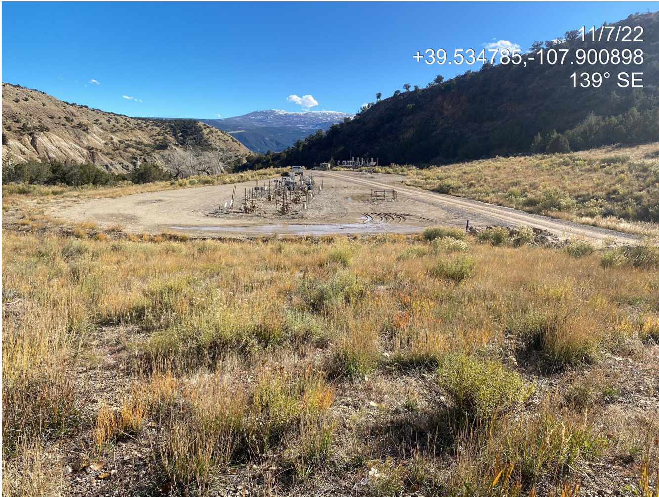
Photo 1. Photo taken from the north shows an overview of the location.
