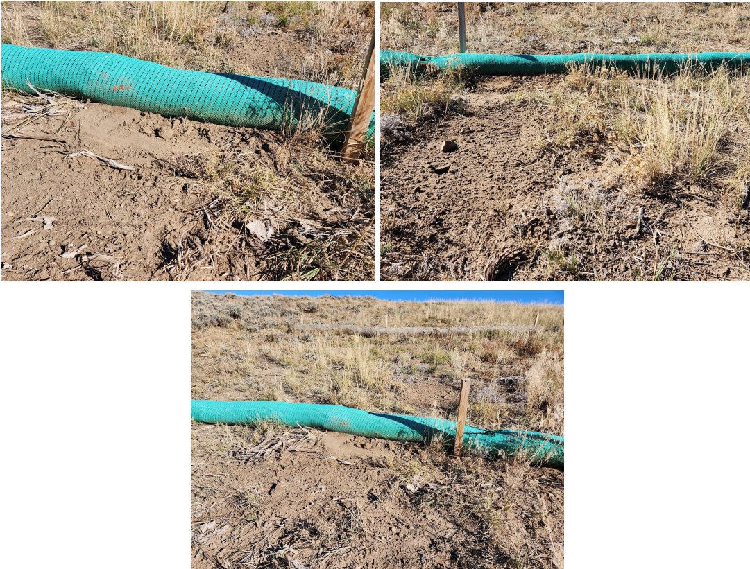
Photos 1-3: Undercutting on wattle repair.
