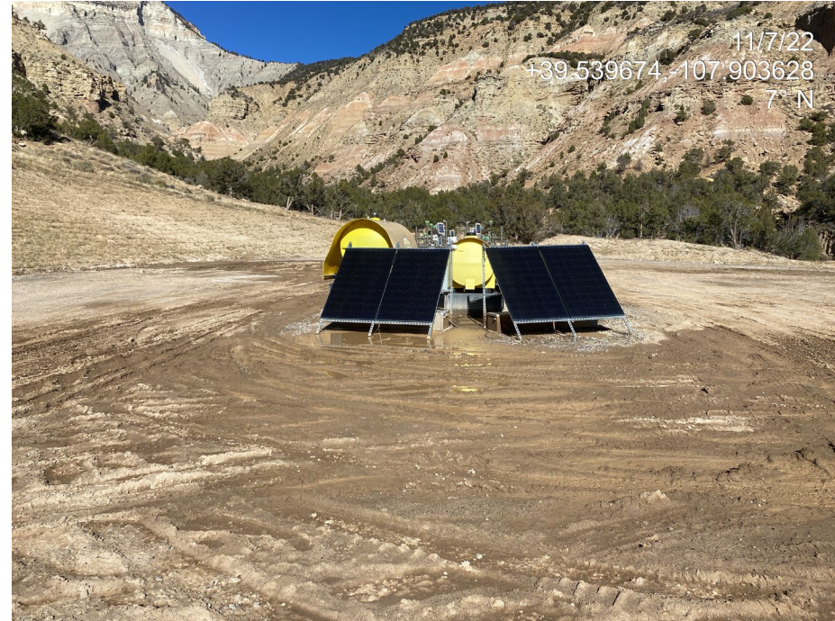
Photo 7. Photos show a lack of stabilization/compaction degradation to the pad surface.
