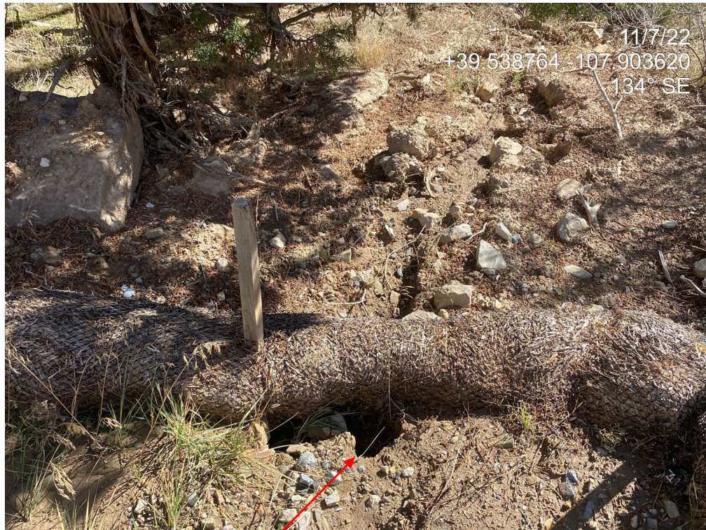
Photo 6. Photos taken at the southeast of the Location shows a wattle installed along the downslope perimeter is not in proper functioning condition; stormwater has cut under the wattle, resulting in offsite degradation.
