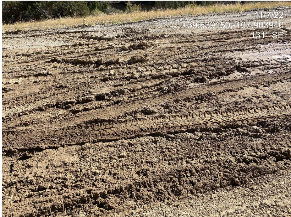
Photo 7. Photos show a lack of stabilization/compaction degradation to the pad surface.
