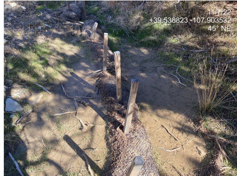
Photo 5. Photo shows where sediment laden stormwater flows have overtopped a wattle at the eastern perimeter of the Location.
