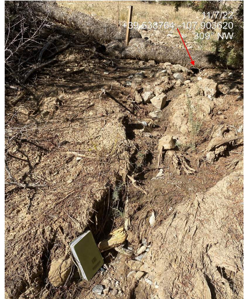
Photo 6. Photos taken at the southeast of the Location shows a wattle installed along the downslope perimeter is not in proper functioning condition; stormwater has cut under the wattle, resulting in offsite degradation.
