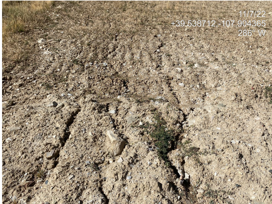
Photo 4. Photo shows a portion of the western interim area, at the base of the slope where erosion degradation is occurring.
