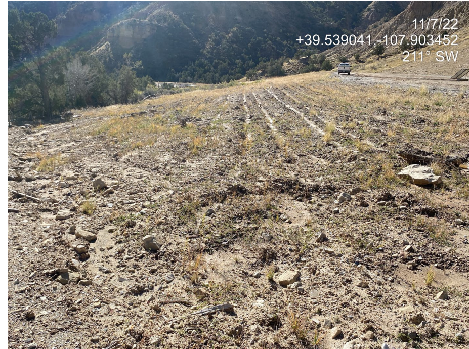
Photo 9. Photo shows interim areas at the east of the Location are overall stable at the time of this inspection. Initial establishment of seeded species is widespread.
