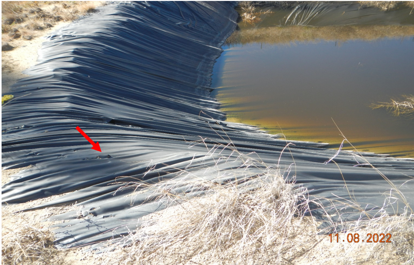
Photo 3. There are holes in the pit liner.
