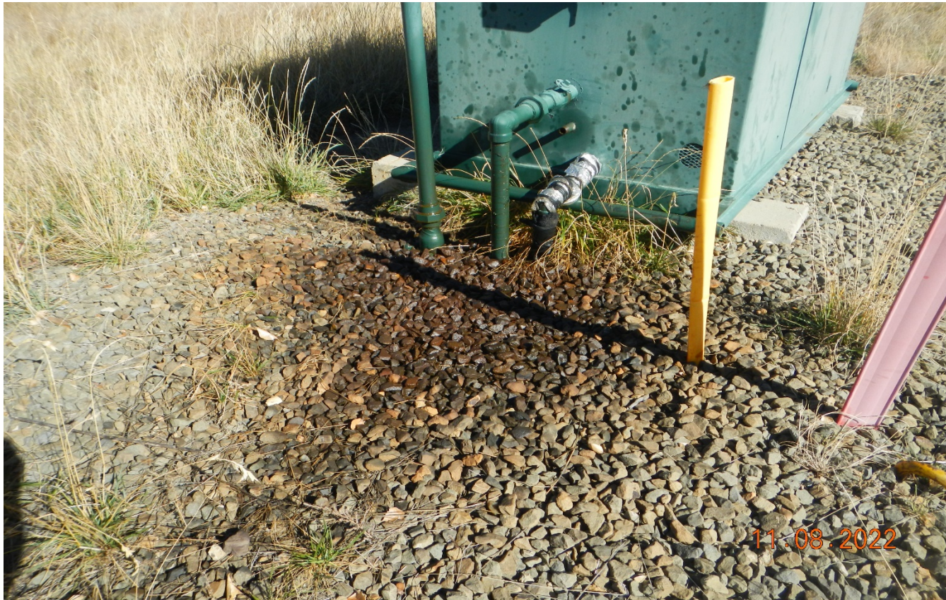
Photo 5. There is stained soils at the meter shed that need to be cleaned up.
