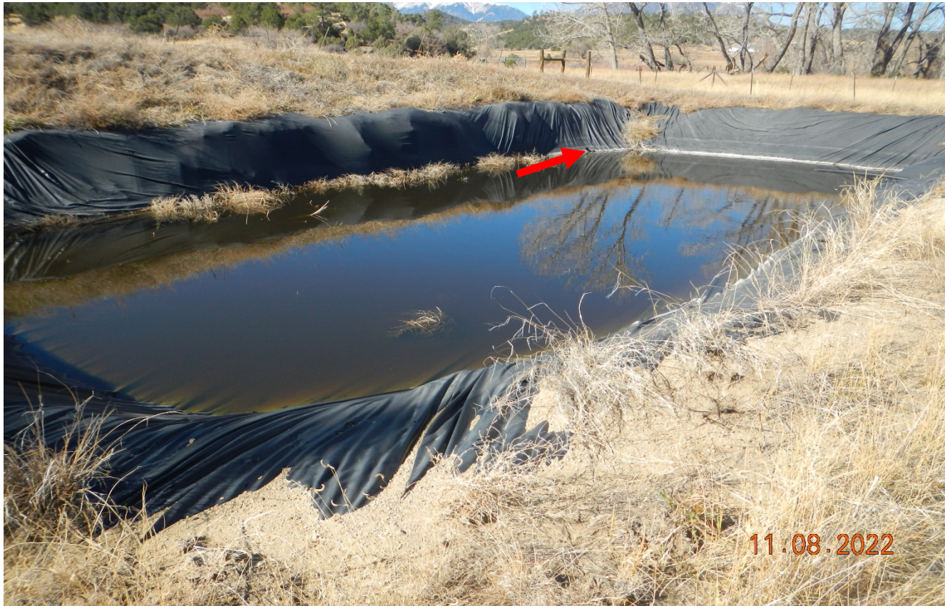
Photo 2. There are holes in the pit liner which need to be replaced.
