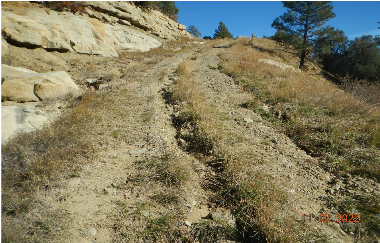
Photo 2. There is erosion channels along this area of access road that need to be repaired.
