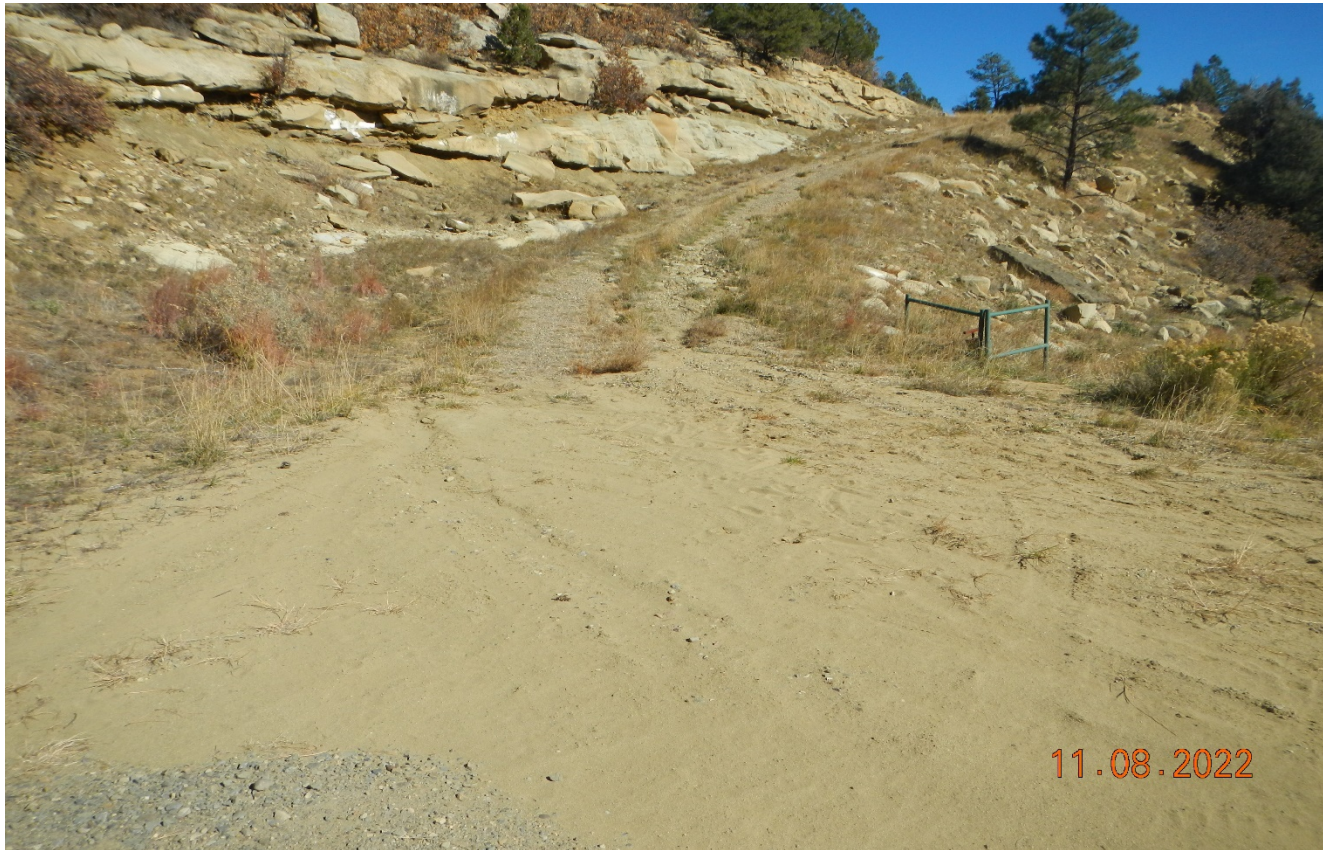
Photo 1. Facing at the beginning of the access road. Sediment is accumulating in this area from erosion of the access road.
