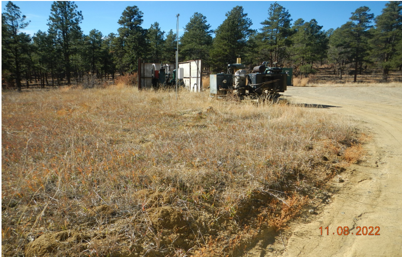
Photo 2. Facing southwest toward the location.
