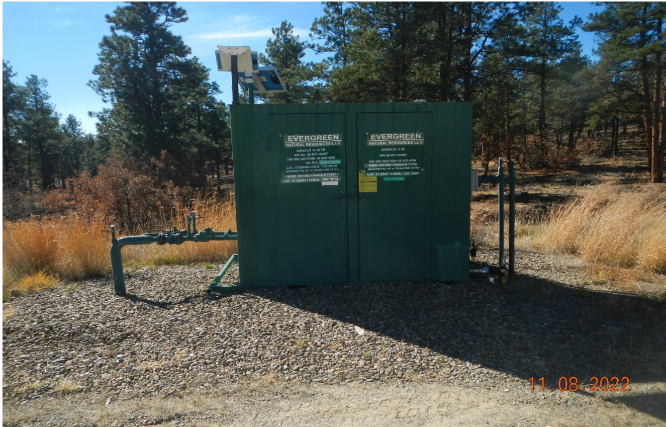
Photo 3. The well signs are posted at the meter shed.
