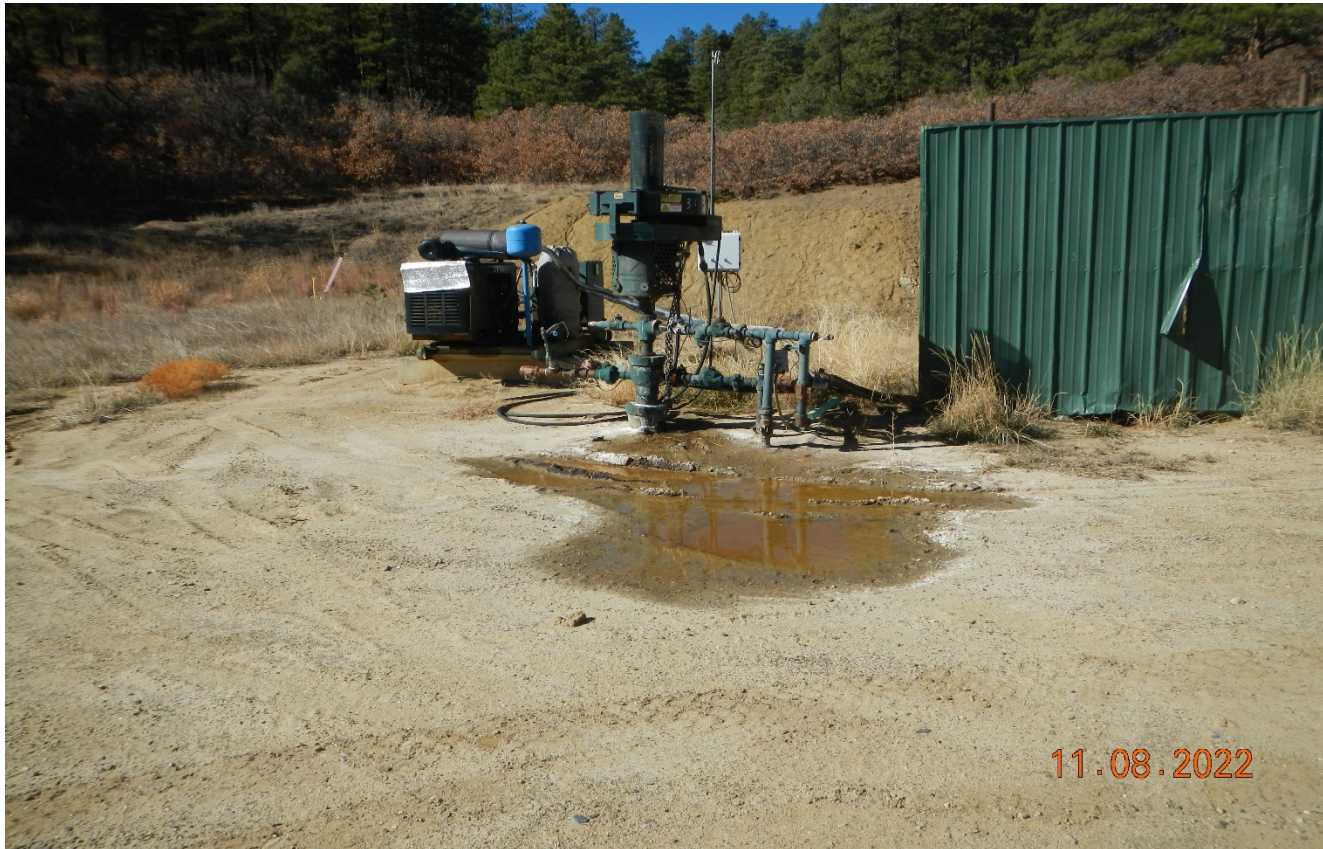
Photo 3. There is dripping water leak at the wellhead that needs to be repaired.
