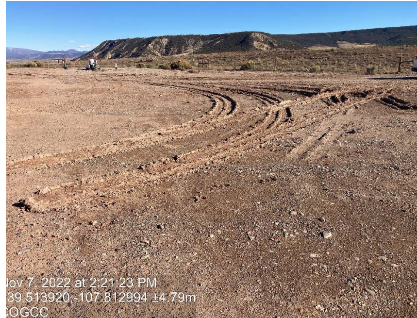
Lack of stabilization/compaction
