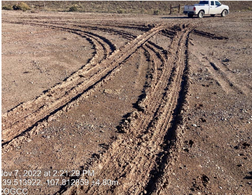
Lack of stabilization/compaction
