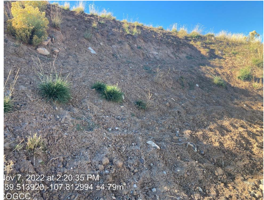
Cut slope lack of stabilization
