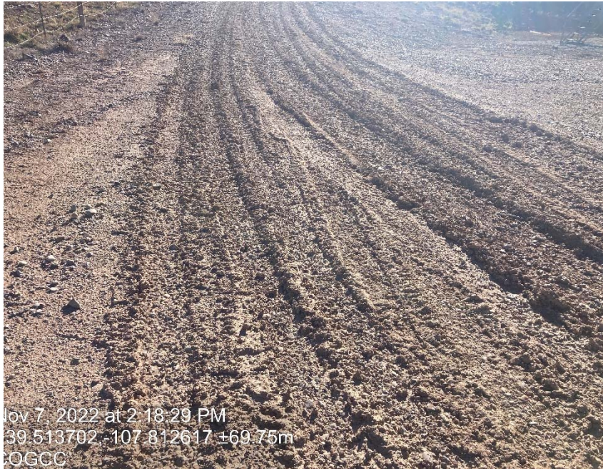
Lack of stabilization/compaction
