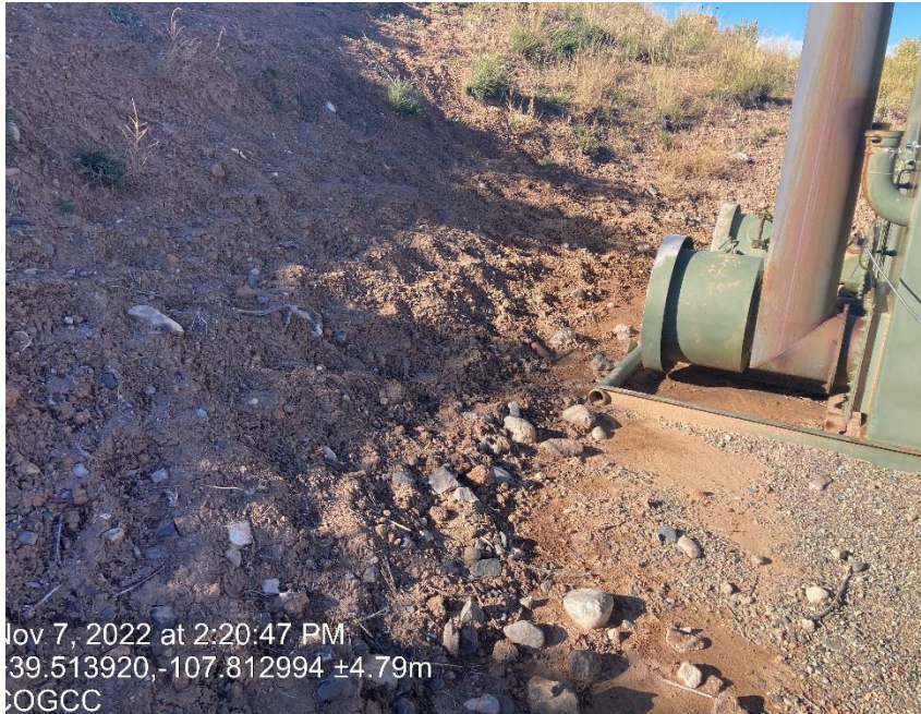
Cut slope lack of stabilization
