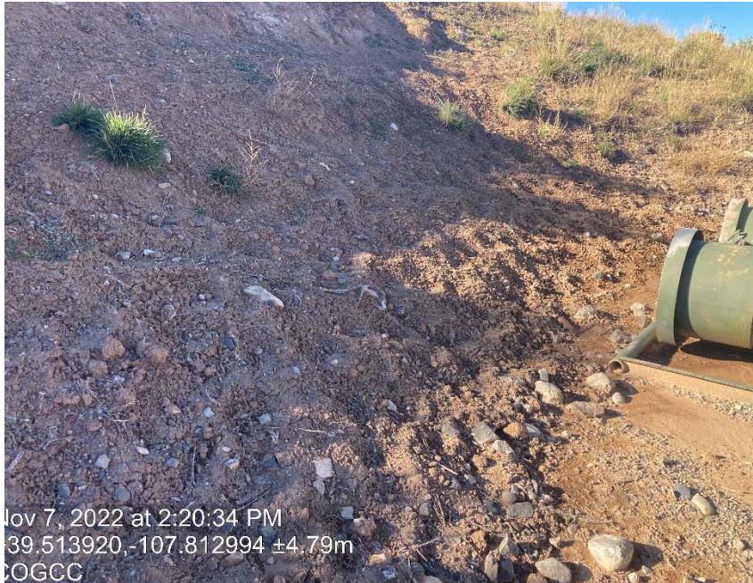
Cut slope lack of stabilization
