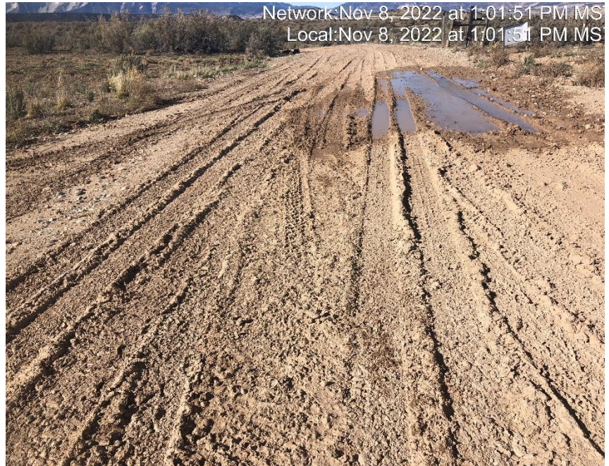
Photo #8337 Insufficient tracking BMP at entrance.
