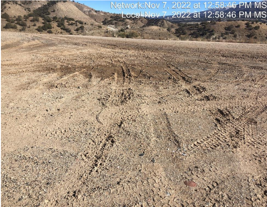
Photo #8321 Insufficient tracking BMP at entrance to location.
