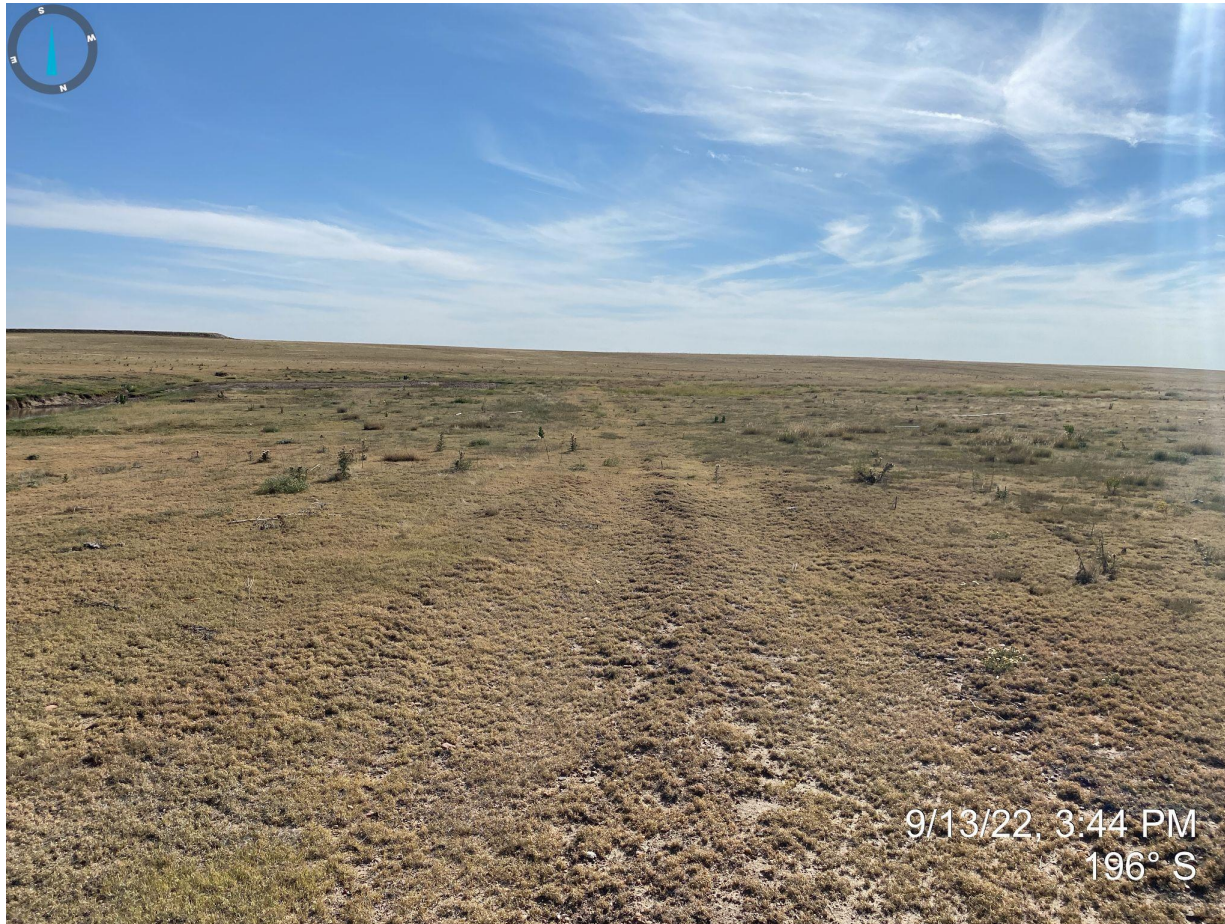
Photo 3. Taken south of the access road “Y intersection”, facing south. Photo illustrates that the location’s access road has minimal contour and grading differences with the adjacent reference areas. The access road also appears to have achieved COGCC final reclamation vegetation standards (e.g. predominantly buffalo grass).
