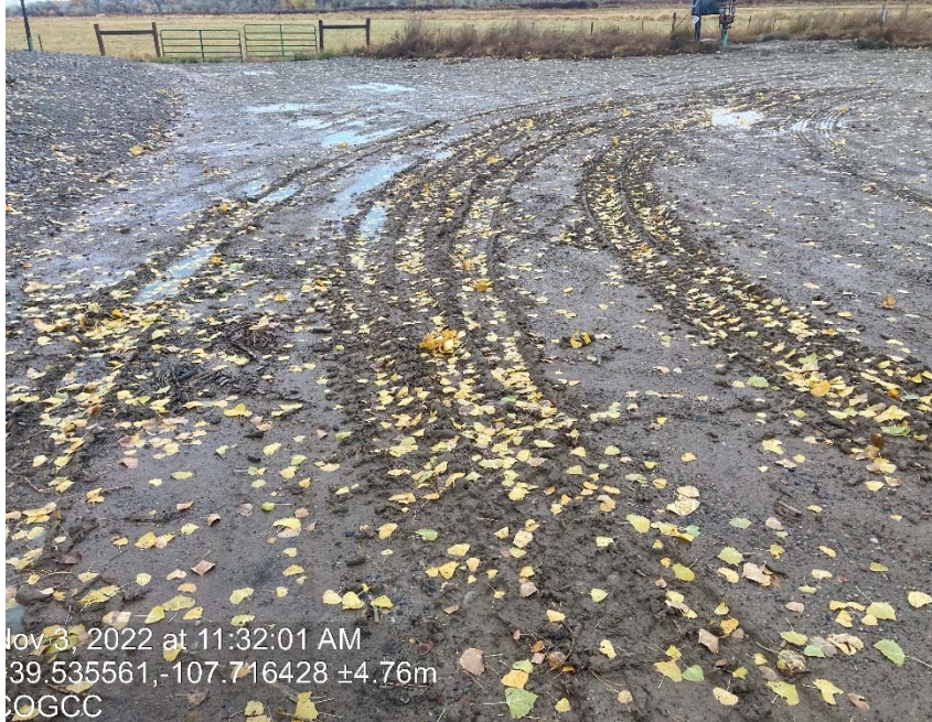
Lack of stabilization/ compaction
