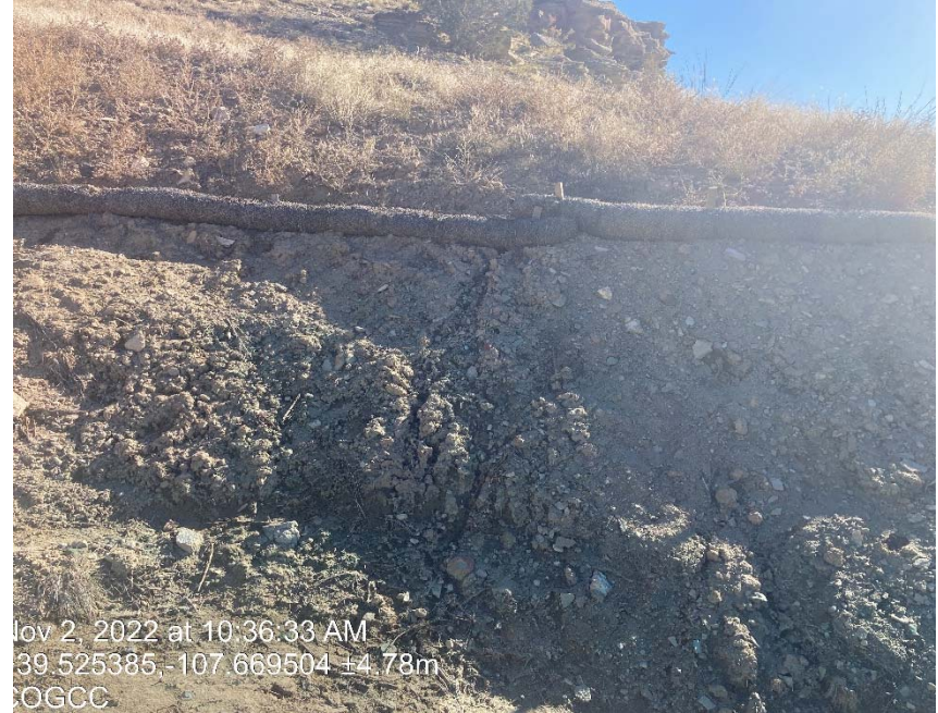
Erosion BMP's Failing
