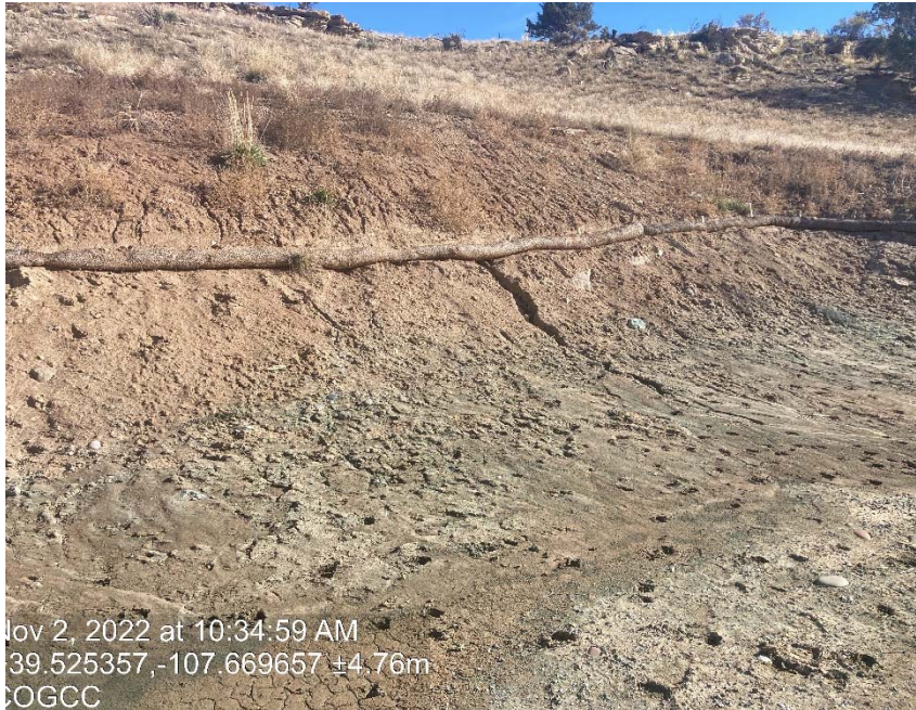
Erosion BMP's Failing
