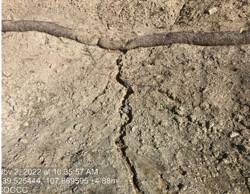
Erosion BMP's Failing
