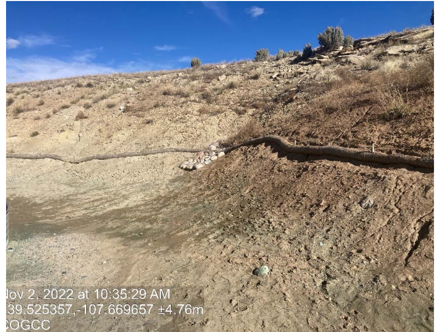
Erosion BMP's Failing
