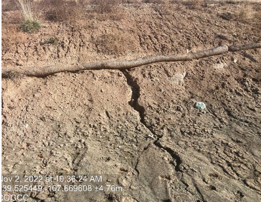
Erosion BMP's Failing
