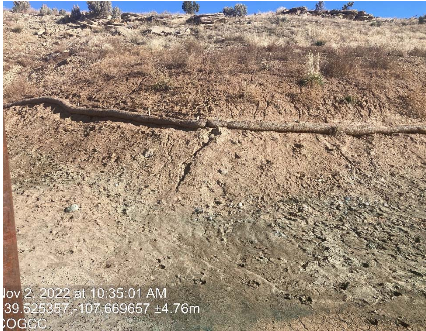
Erosion BMP's Failing
