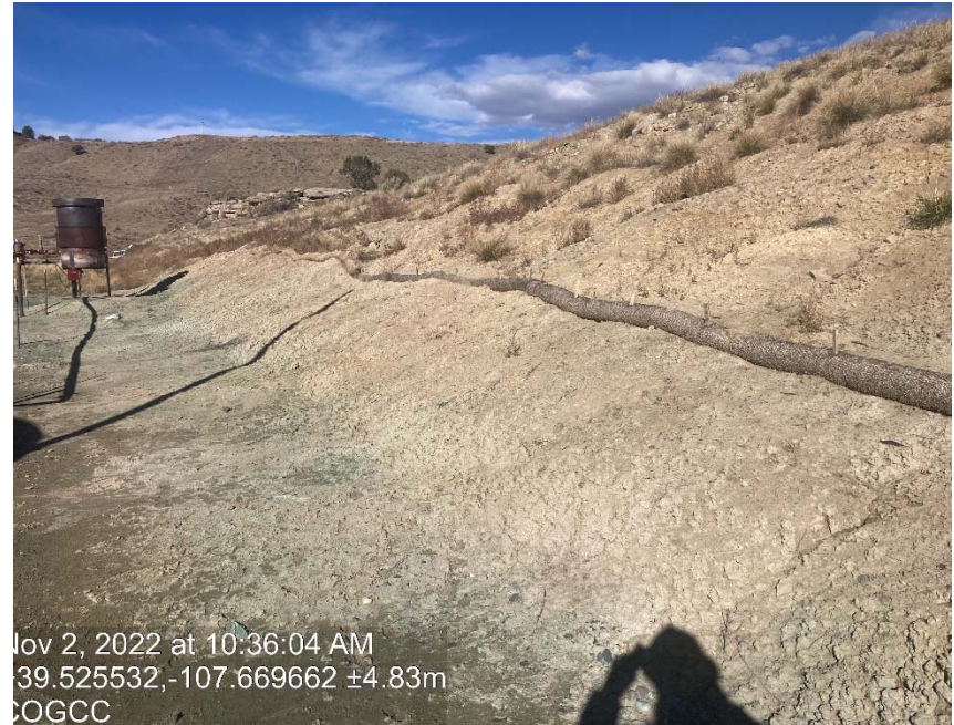
Erosion BMP's Failing
