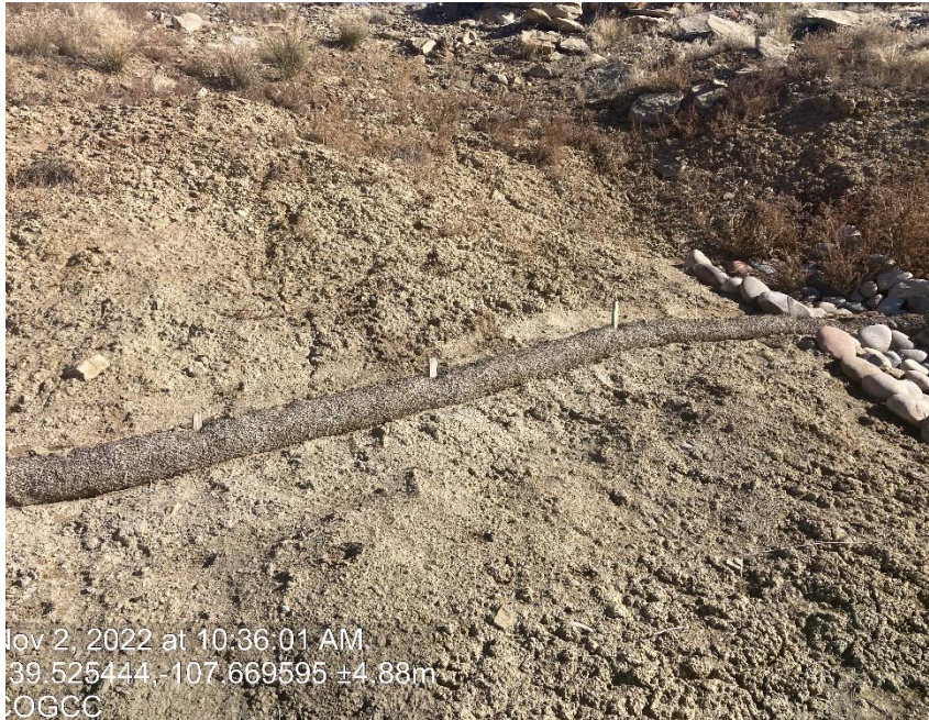
Erosion BMP's Failing
