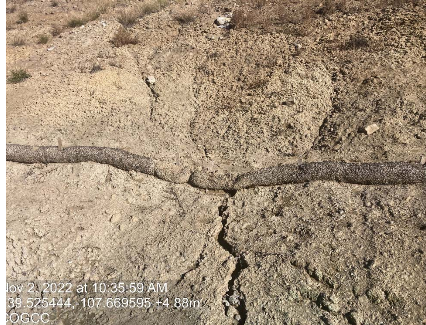
Erosion BMP's Failing
