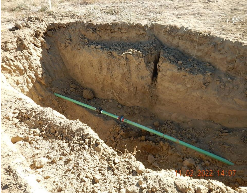
Isolation valve installed on MSSU 19-5 flowline adjacent to/ west of Krauss Battery. Valve can to be installed for access.
