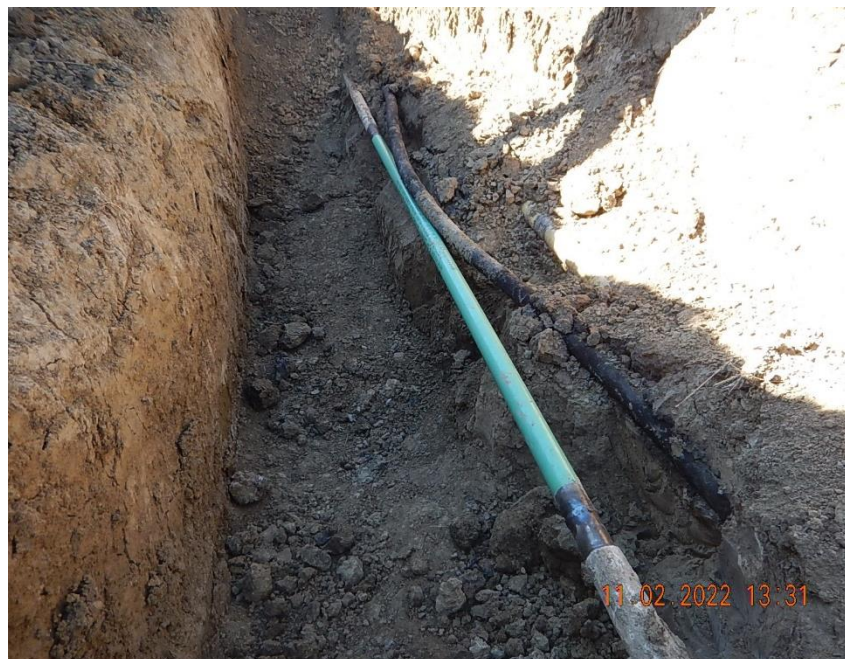
View of flowlines exposed in excavation at release point. (1) 2" carbon steel flowline repaired; approximately 15' of 2" CS FBE coated pipe welded into place (welds to be coated) in area of failure. (1) poly natural gas flowline running tandem in same trench.
