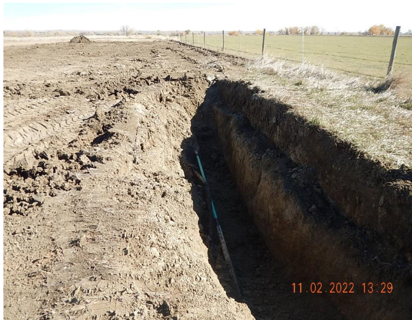
Flowlines exposed in excavation; repair completed on produced water injection flowline. View east toward MSSU 19-5 injection well. Located at approx 40.648722, -105.049226
