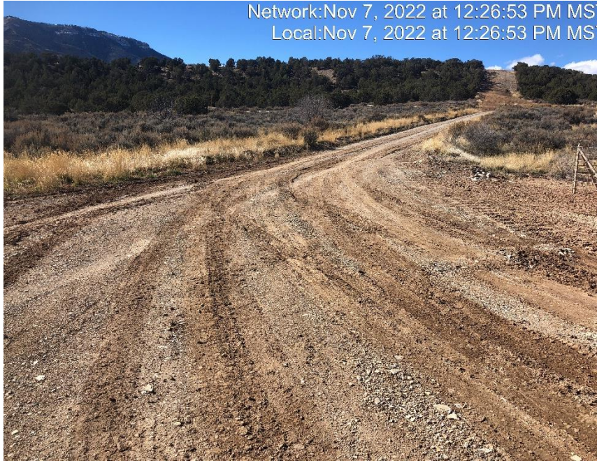
Photo #8308 Insufficient tracking BMP at entrance to location.
