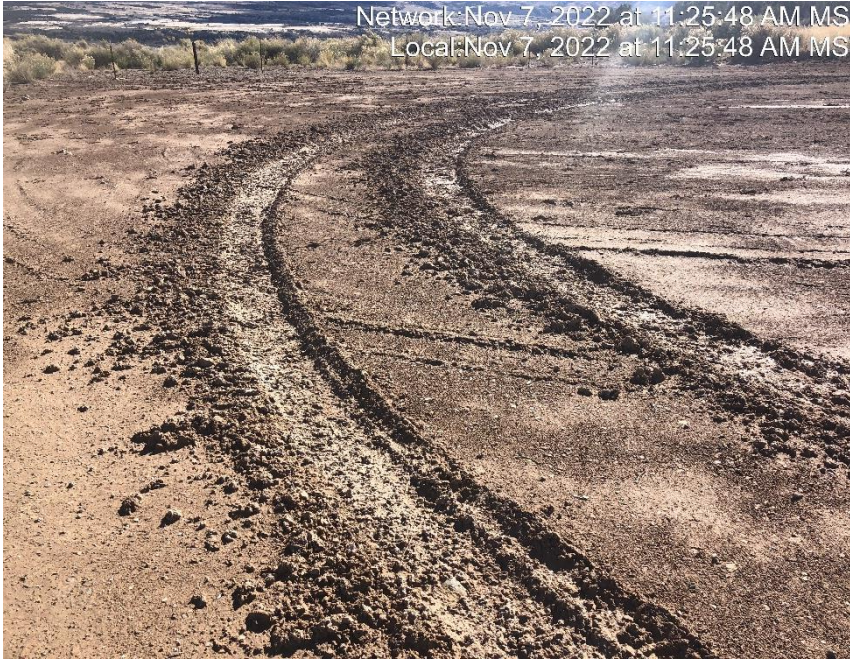
Photo #8298 Location lacks stabilization.
