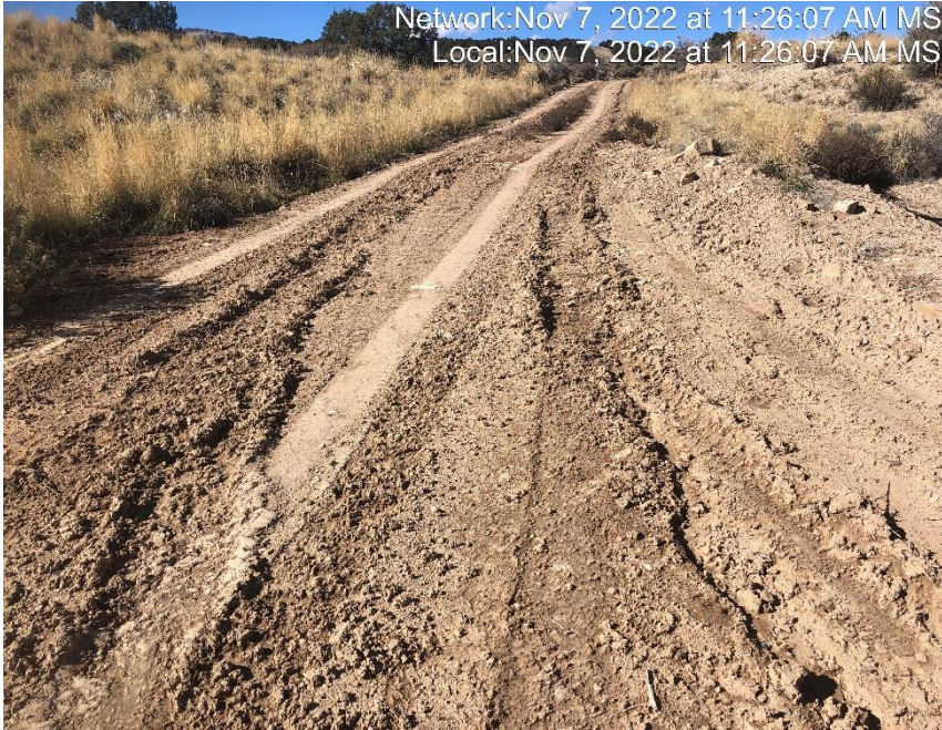
Photo #8300 Insufficient tracking BMP at entrance to location.
