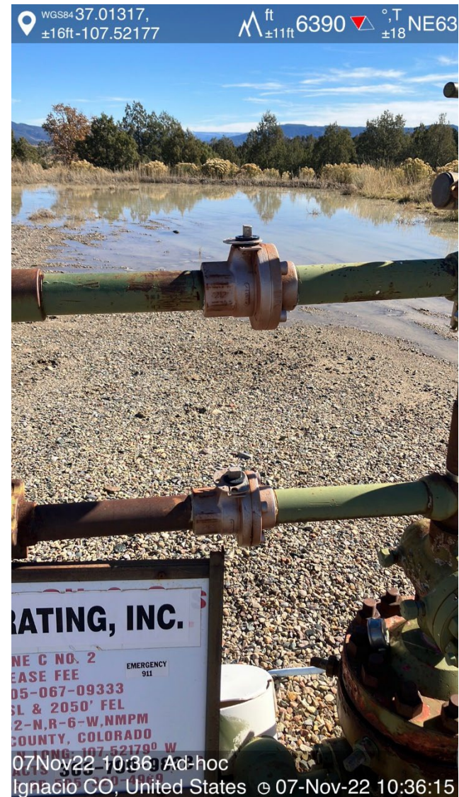
IMG 04 C-2 wellhead, lower valve open
