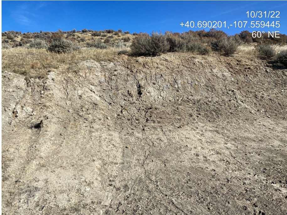
Photo 6. Photo shows the cut slope at the northeast of the Location is bare and unprotected. Rill erosion is evident throughout unvegetated portions of cut slopes.
