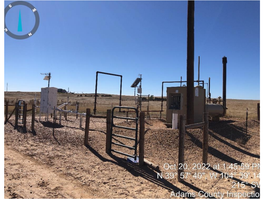
Photo#2 Separator and meter run.
