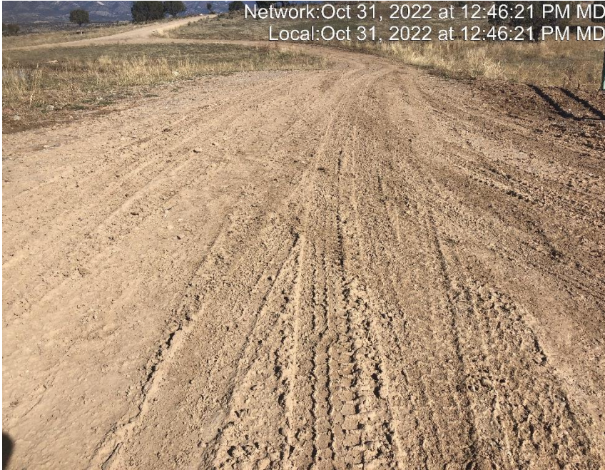
Photo #8272 Insufficient tracking BMP at entrance to location.
