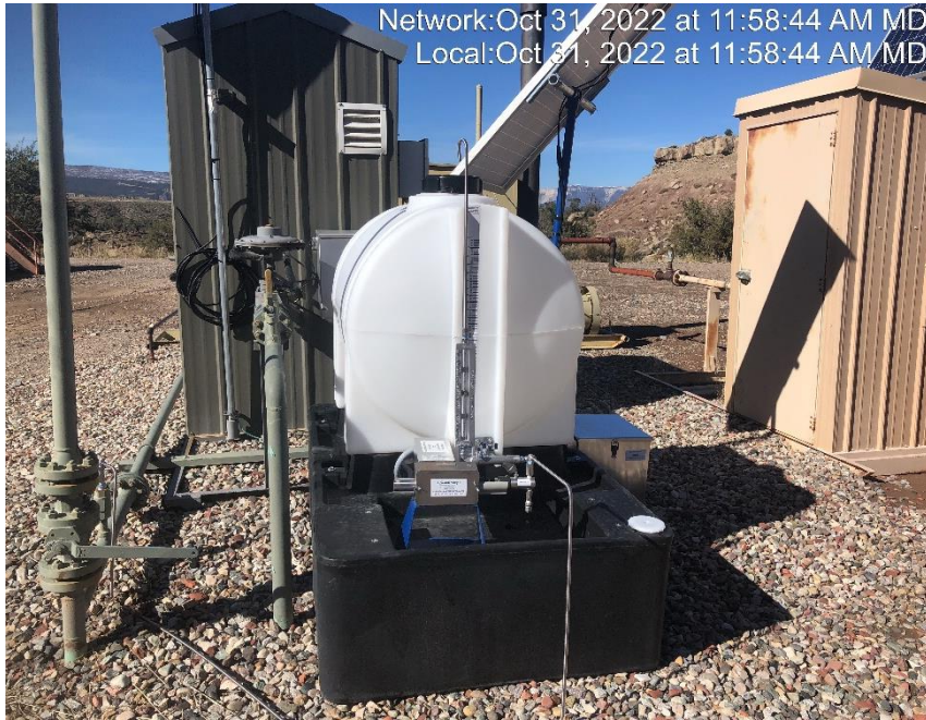
Photo #8252 Chemical tank missing required information.
