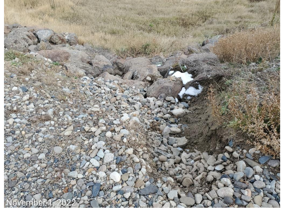
Photo 2: Photos taken from the north end of the Location, at the location entrance. Photo shows stormwater runoff has resulted in erosion degradation to the slopes. BMPS missing or insufficient.
