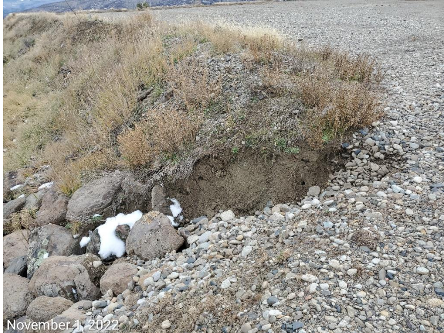
Photo 2: Photos taken from the north end of the Location, at the location entrance. Photo shows stormwater runoff has resulted in erosion degradation to the slopes. BMPS missing or insufficient.
