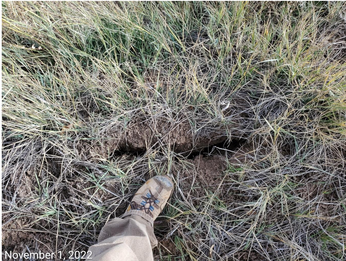
Photo 5: Photo taken from the perimeter berm on the southeast end of the Location. Photo shows cracks along the perimeter of the location are beginning to re-develop.
