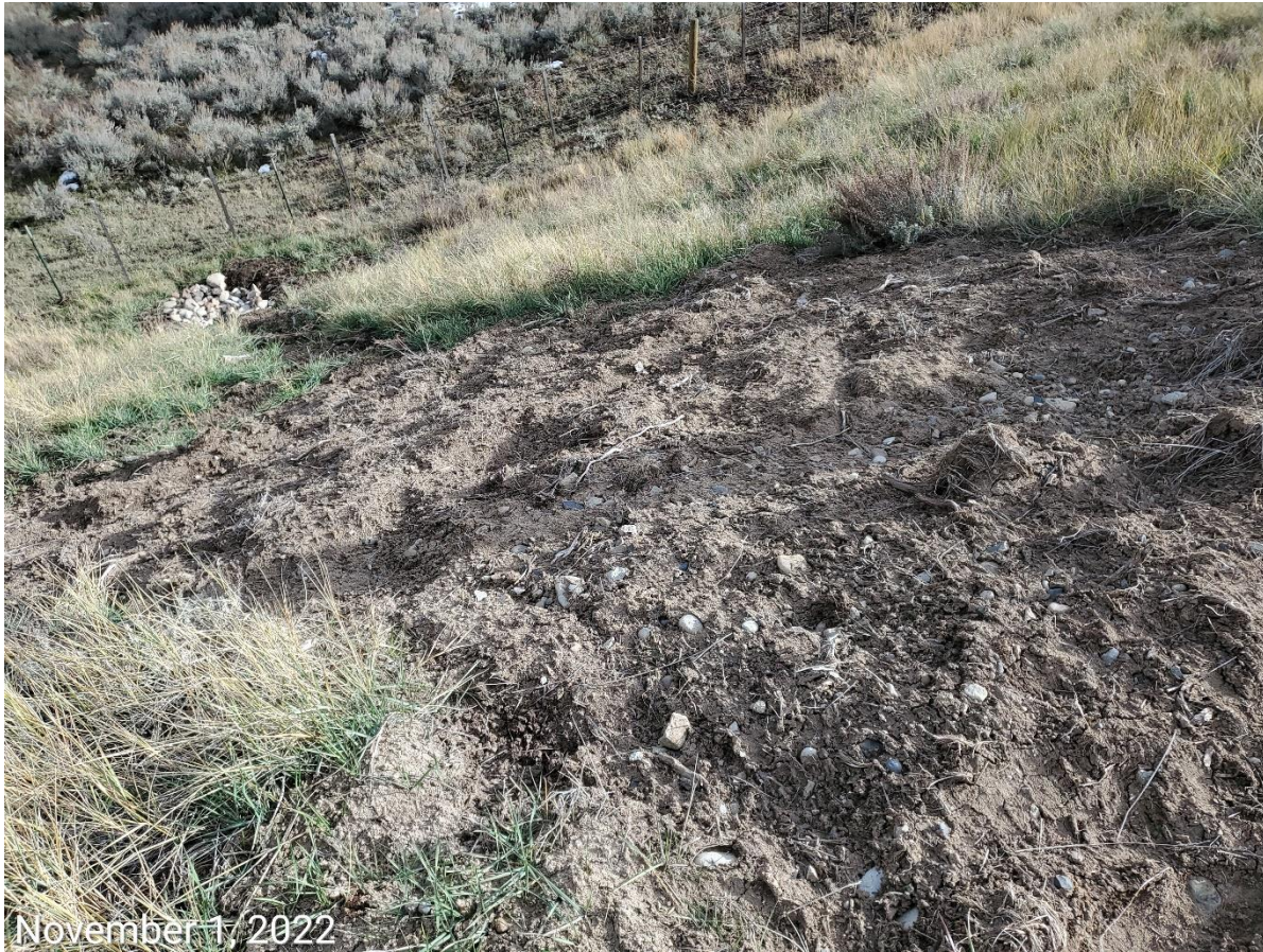
Photo 3: Photo taken from the southeast end of the Location. Photo shows areas where Operator appears to have installed a slope drain. Soils on the slopes have been left bare and at risk to erosion degradation.
