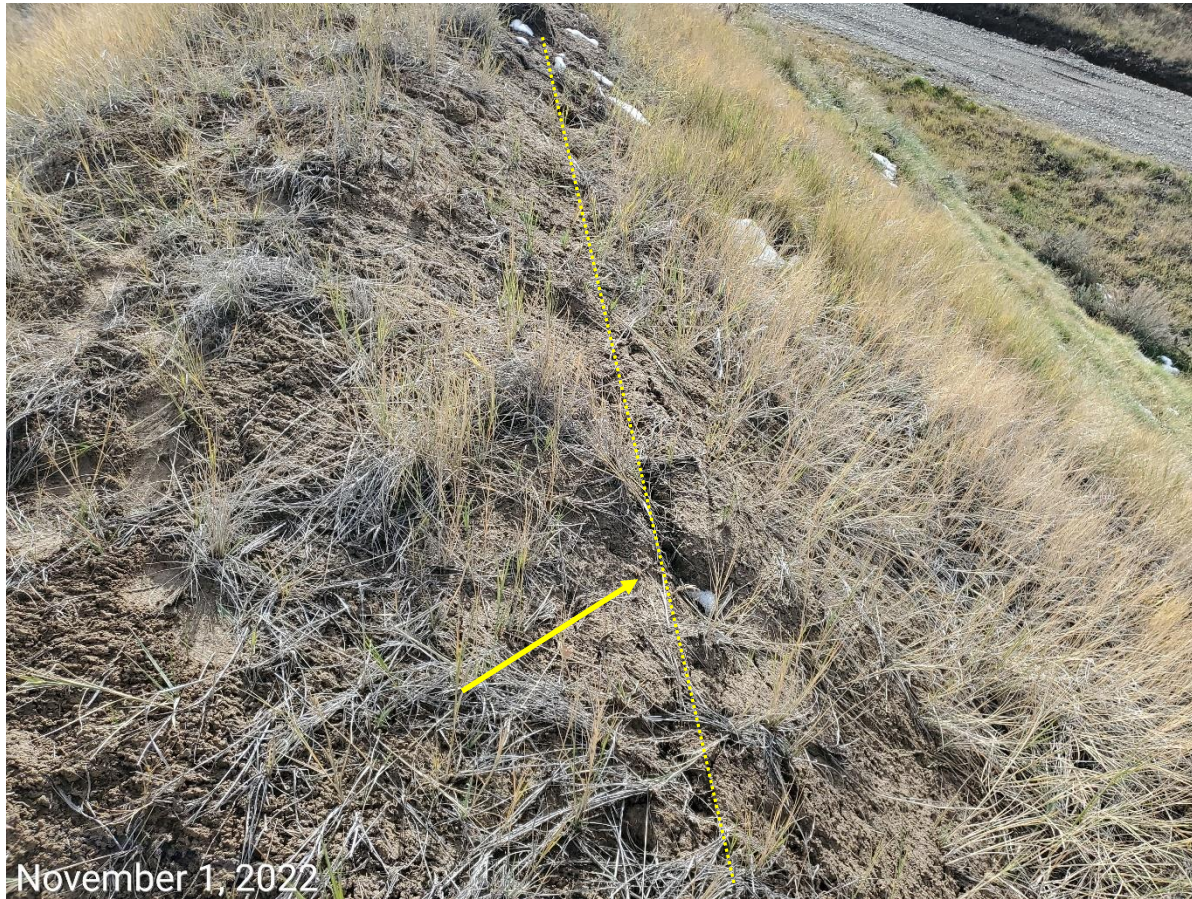
Photo 4: Photo taken from the perimeter berm on the northwest end of the Location. Photo shows cracks along the perimeter of the location are beginning to re-develop.
