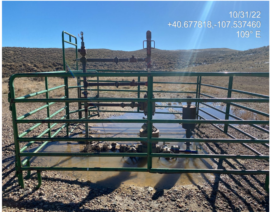
Photo 6. Photo shows the wellhead. Wellhead signage does not comply with Rule 605.d; API number not present.
