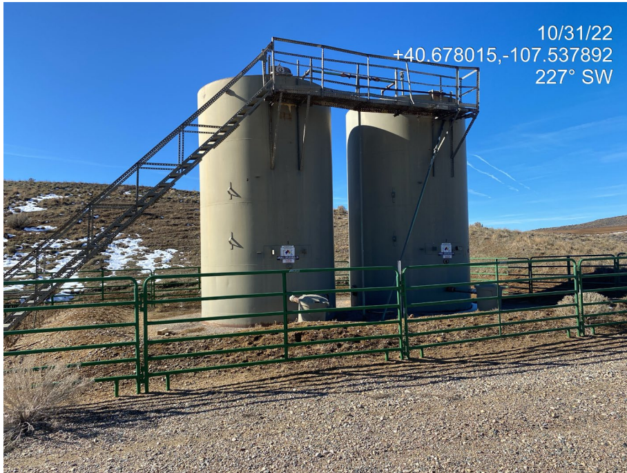
Photo 2. Photo taken from the southwest shows the tank battery signage is missing/insufficient.
