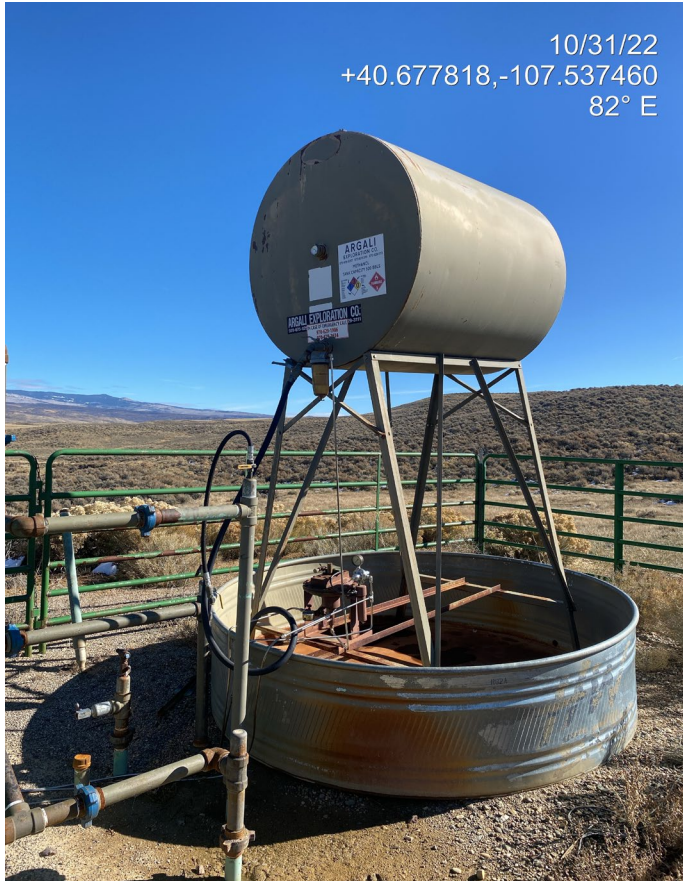
Photo 5. Photo taken from the northeast. The methanol tank secondary containment lacks wildlife protection BMPs. The tank label is inaccurate; tank capacity reads 500 BBLS.
