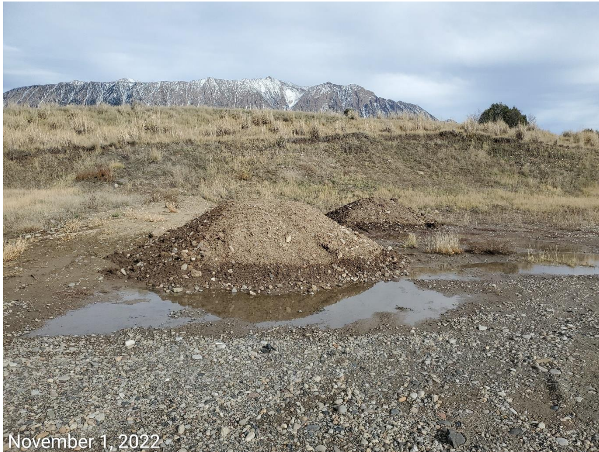
Photo 3: Photo taken from the north end of the Location. Photo shows soils stockpiles with missing BMPs to protect stockpiles from wind and water erosion, as well as to minimize erosion, degradation and sediment transport
