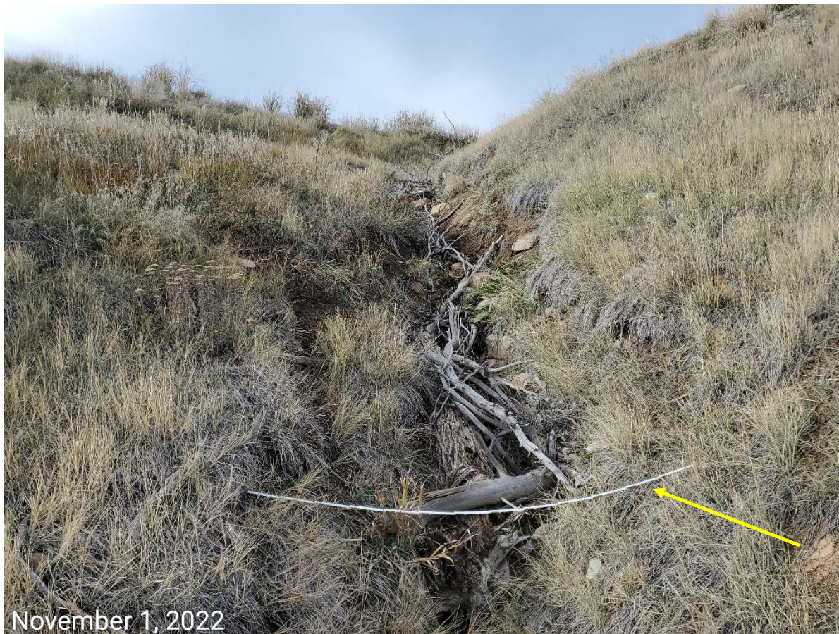
Photo 8: Photo taken from the northern inlet at the sediment trap on the east end of the Location. Photos shows sediment trap has not been constructed with a properly engineered inlet per corrective actions; gully erosion due to stormwater runoff into trap remains evident. 6 and ½ foot measuring stick used for scale (arrow).
