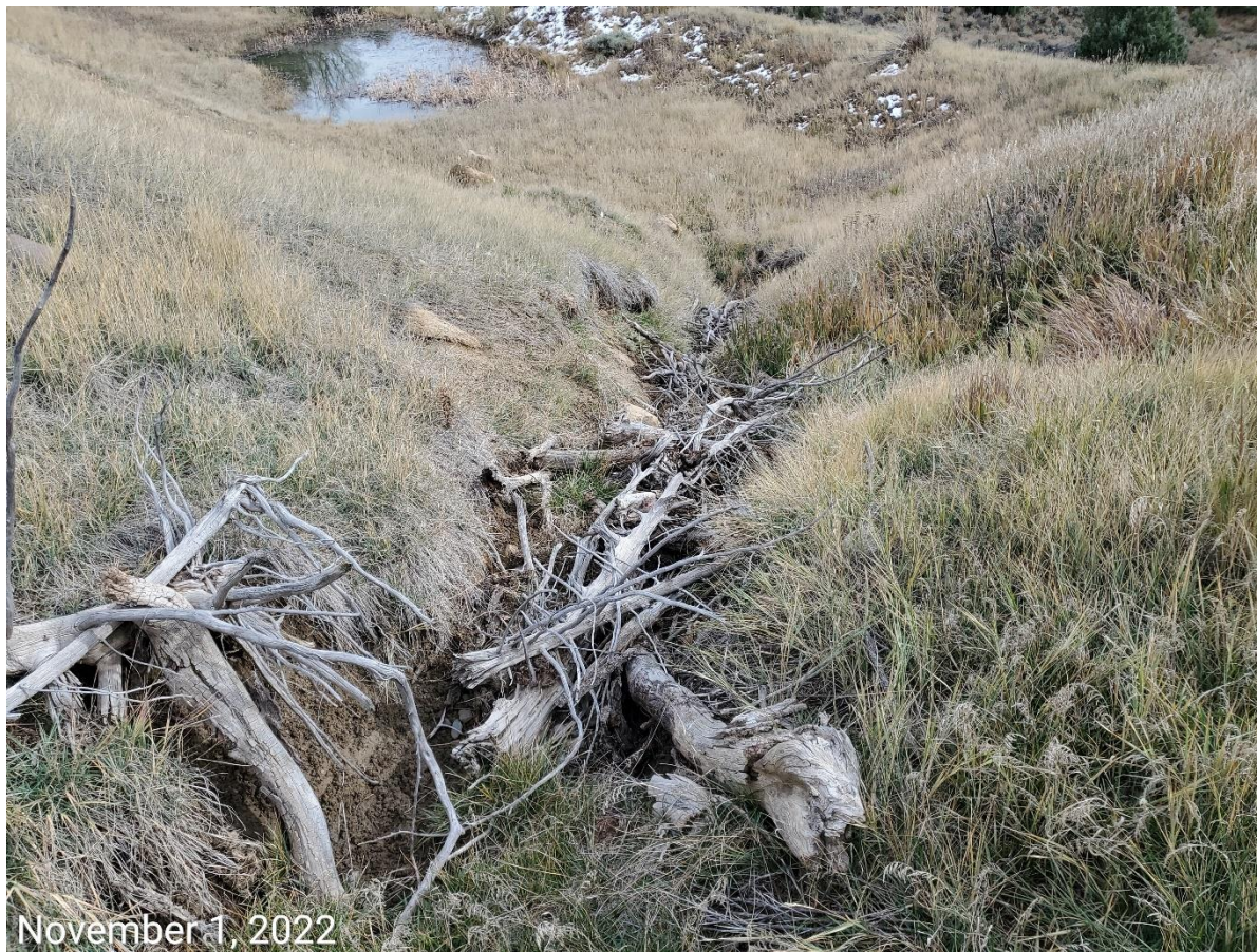
Photo 6: Photo taken from the northern inlet at the sediment trap on the east end of the Location. Photos shows sediment trap has not been constructed with a properly engineered inlet per corrective actions; gully erosion due to stormwater runoff into trap remains evident.
