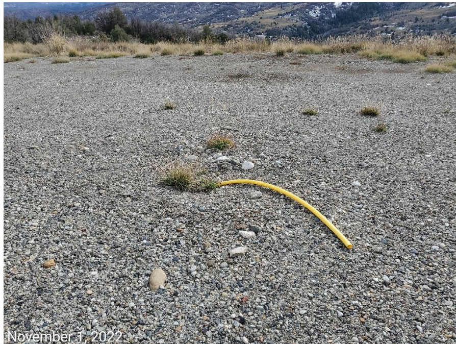
Photo 11: Photos examples showing markers at anchors not in proper functioning condition. Maintenance required. Unable to find anchor associated with marker observed in left photo.
