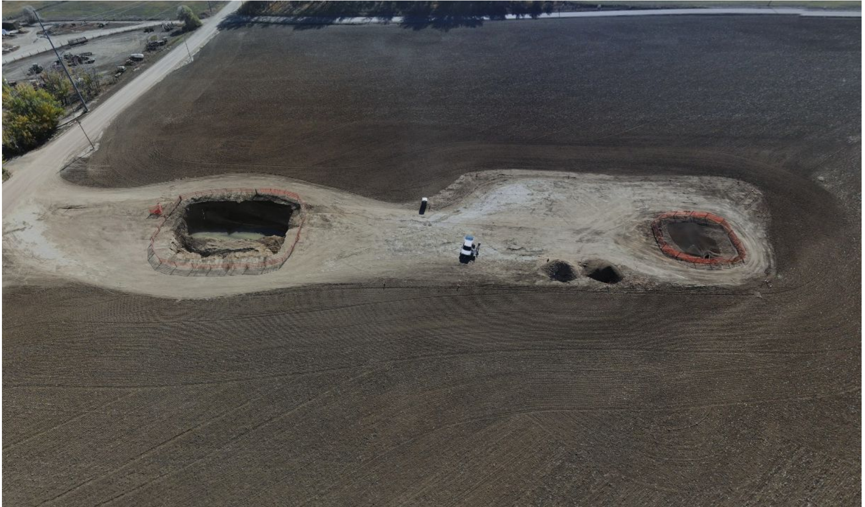
Photo 2. COGCC drone aerial imagery taken on 11/2/2022 illustrating the active remediation projects related to the Halverson 1 well. Photo illustrates an open remediation for the wellhead and tank battery. Photo illustrates the adjacent cropland is fallow and will likely go back into crop production next Spring.
