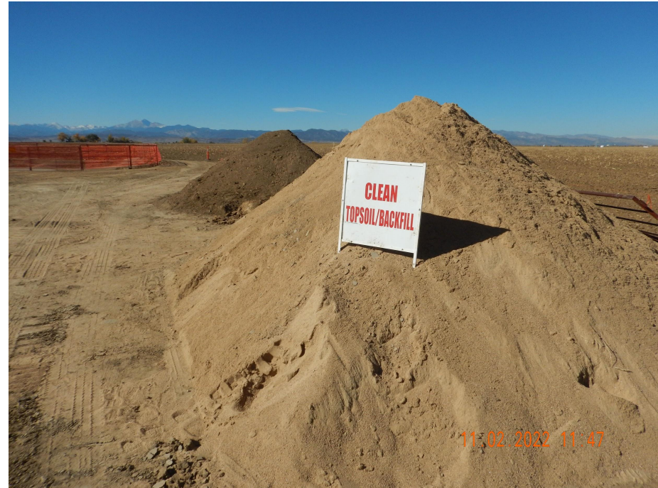
Photo 8. Photo taken from the north central location, facing West. Photo illustrates a stockpile of sand, not topsoil.
