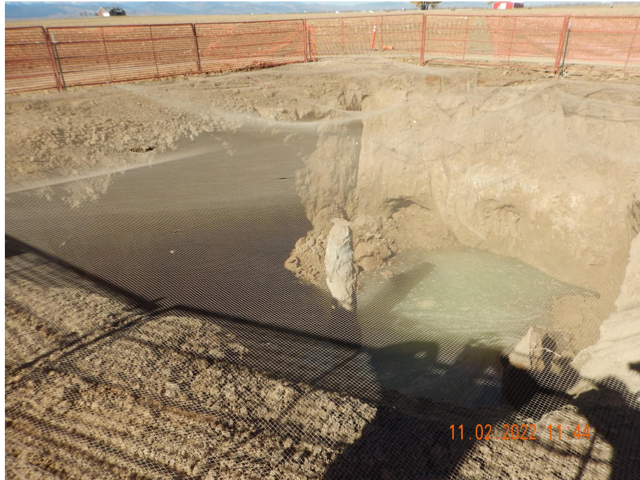
Photo 7. Photo taken from the wellhead excavation, facing Northwest. Photo illustrates netting over the excavation.
