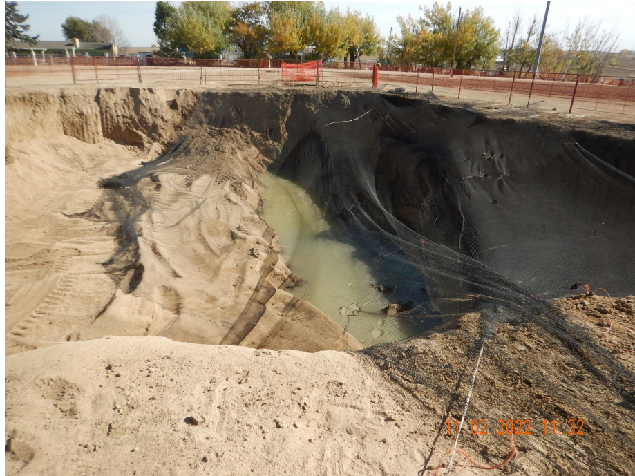
Photo 5. Photo taken from the tank battery excavation, facing East. Photo illustrates netting over the groundwater portion and sand to the north of the groundwater.
