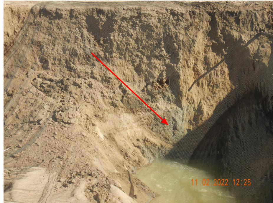
Photo 6. Photo taken of the eastern tank battery sidewall. Photo illustrates sidewall impacts appear to be evident.
