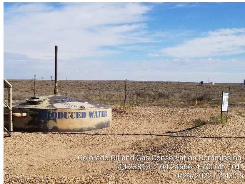
Photo 4 – Produced Water Tank
