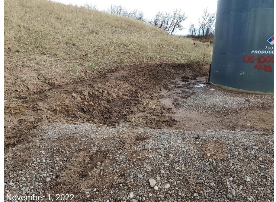
Photo 2: Photos show secondary containment BMPs at the tank battery have been installed or repaired.
