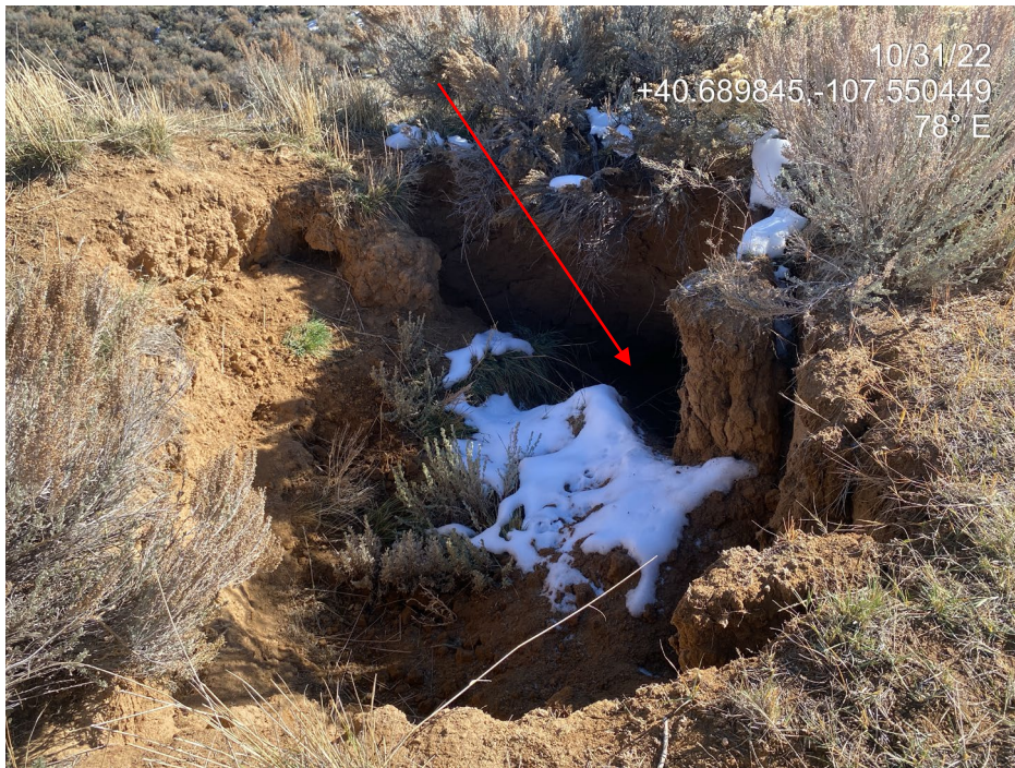
Photo 5. Photo shows erosion occurring in the fill slope at the east of the Location. The hole was approximately 8 by 9 feet wide and 3 feet deep. Arrow indicates the deepest part of the hole which was approximately 10 feet deep.
