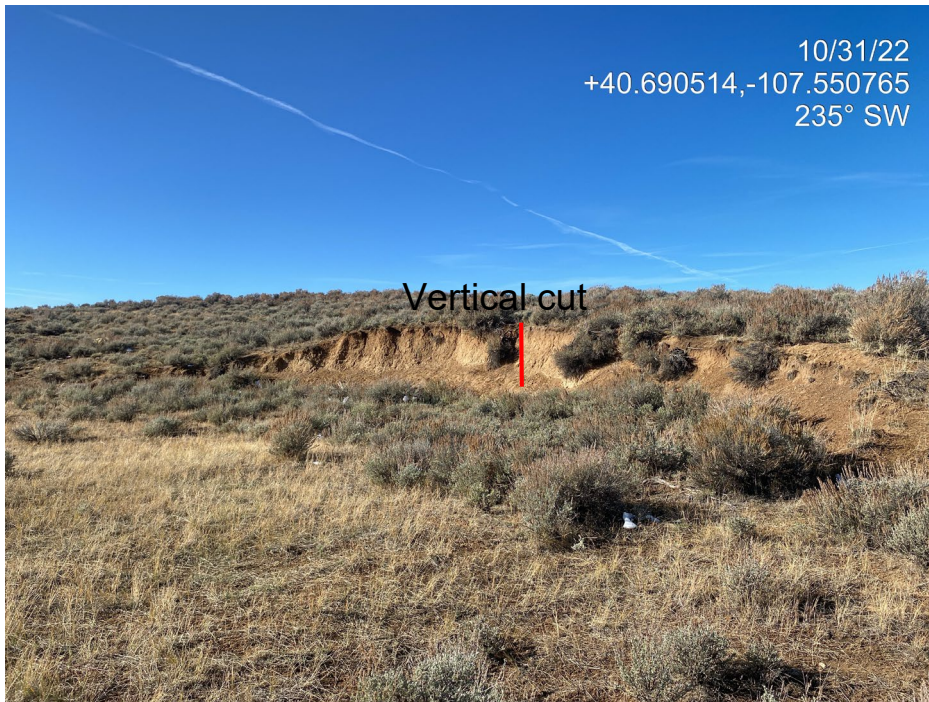
Photo 3. Photo taken from the northwest of the Location shows the cut slope has not been properly reclaimed; vertical cut must be recontoured to match the surrounding landscape and stabilized to prevent erosion.
