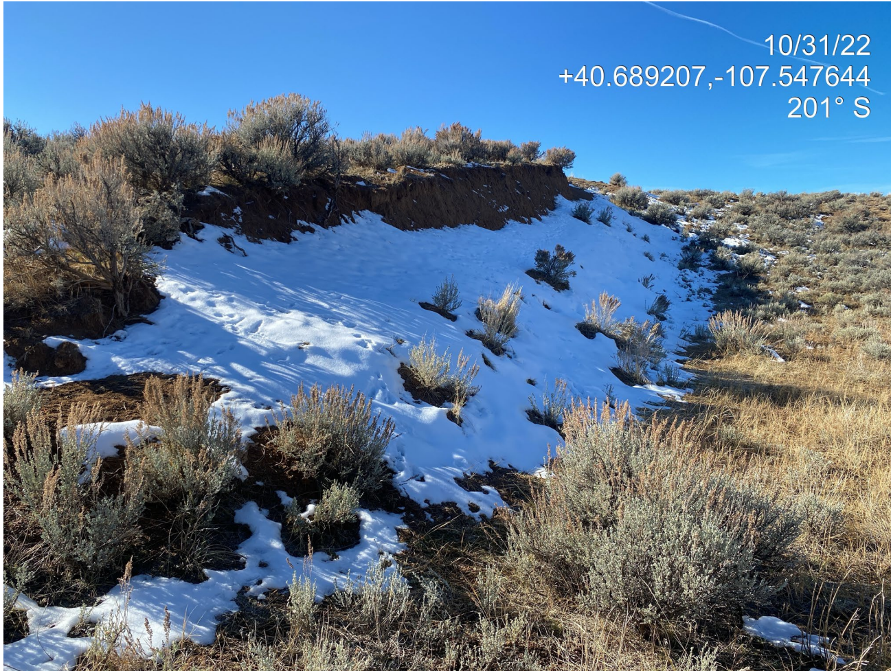
Photo 2. Photo taken from the southwest of the Location shows the cut slope has not been properly reclaimed; vertical cut must be recontoured to match the surrounding landscape and stabilized to prevent erosion.
