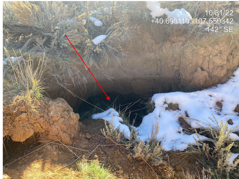
Photo 6. Photo shows erosion occurring in the fill slope at the east of the Location. Arrow indicates the deepest part of the hole which was approximately 10 feet deep.
