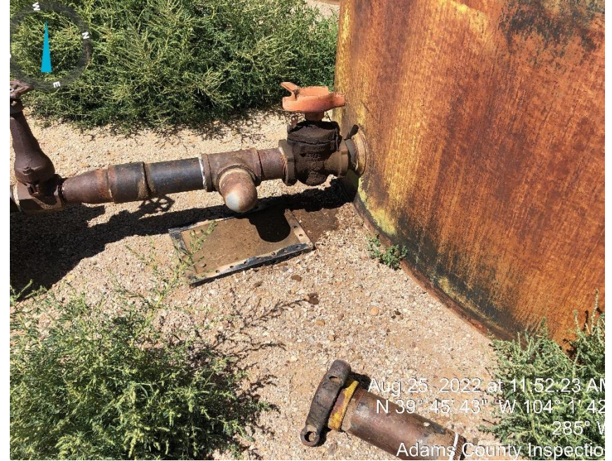
Photo#4. Stained soil under valve on oil tank.
