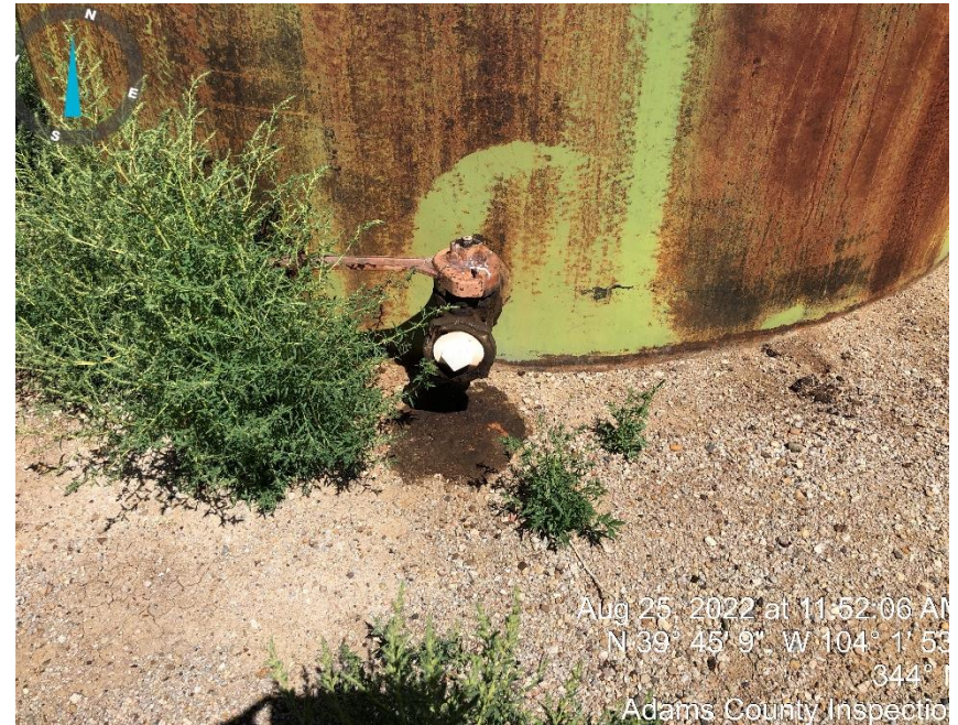
Photo#2. Stained soil under crude tank.
