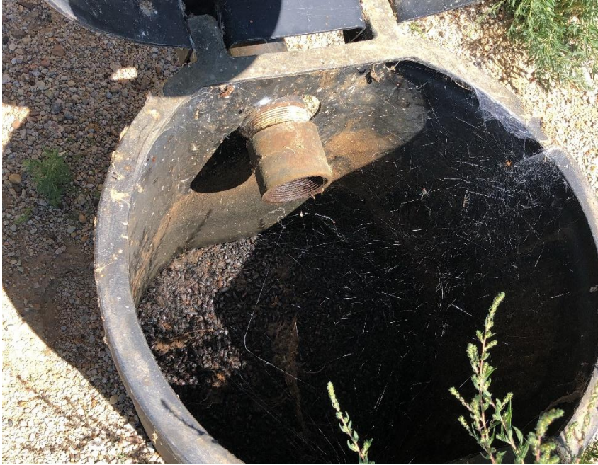
Photo#3. No bull plug in load out bucket.
