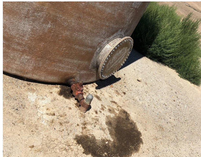
Photo#6. Stained soil on back side of P/W tank.
