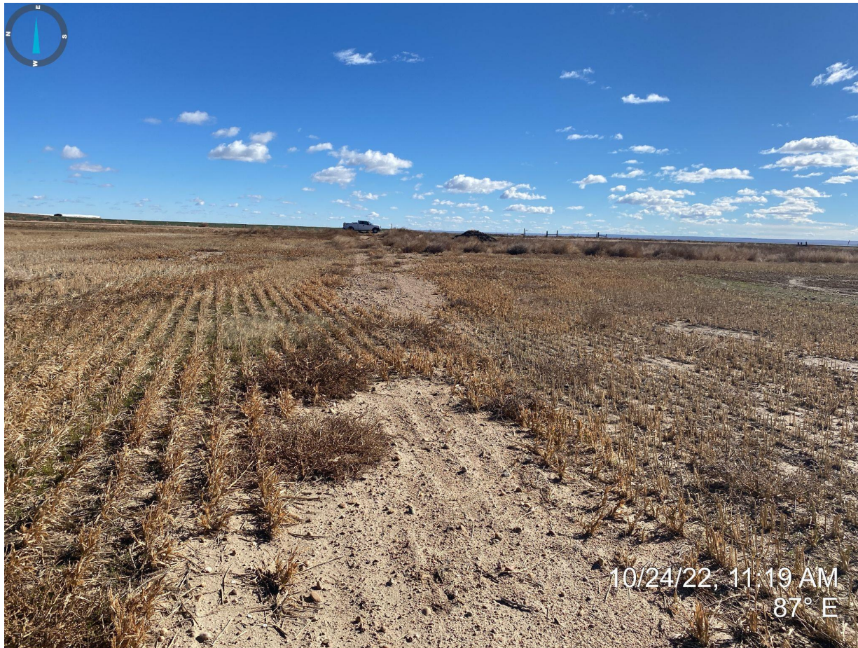
Photo 5. Taken between well and location, facing east. Photo shows access road has not been reclaimed with no evidence of decompaction, gravel/road base present, and non-uniform vegetation cover.
