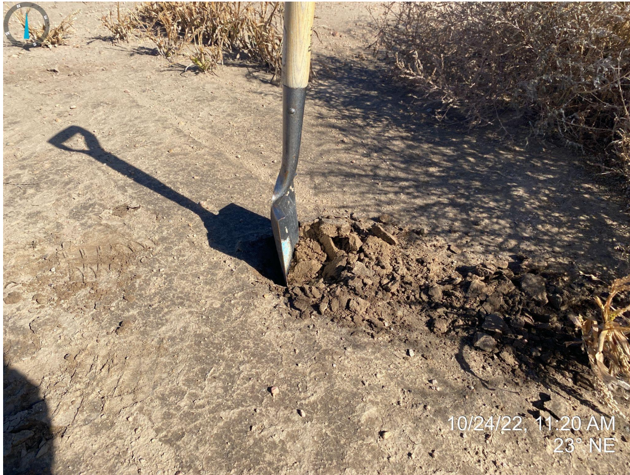
Photo 6. Close up photo taken from pit area. Photo shows the location was not properly decompacted.
