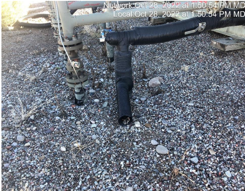
Photo #8228 Flowline insulation open ended and not capped.
