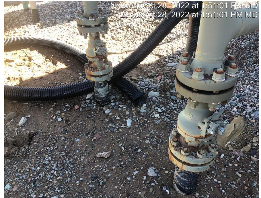
Photo #8229 Flowline insulation open ended and not capped.
