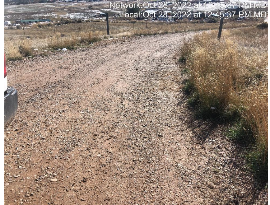
Photo #8224 Insufficient tracking BMP at entrance to location.
