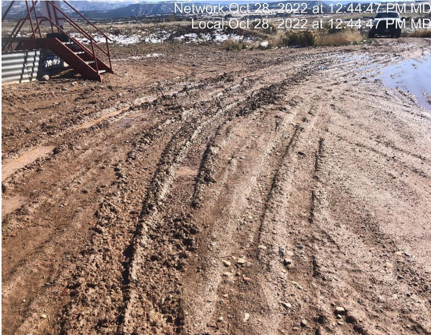
Photo #8222 Location lacks stabilization.
