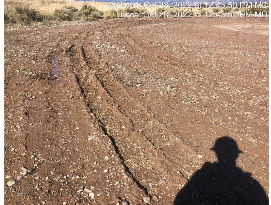
Photo #8219 Location lacks stabilization.
