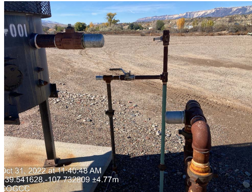
Pipping from tanks to stored equipment disconnected
