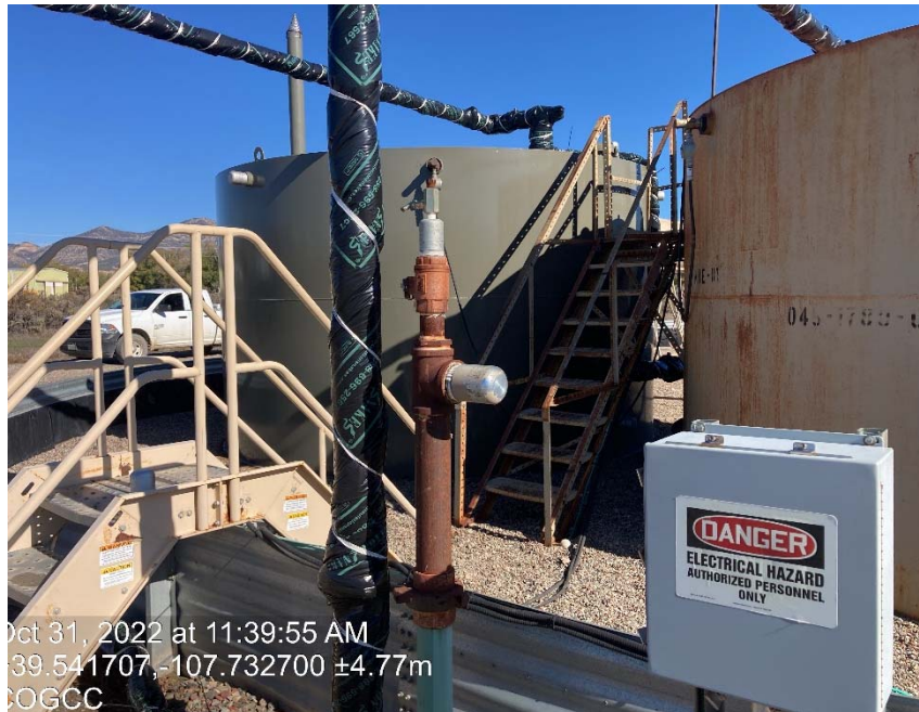
Pipping from tanks to stored equipment disconnected
