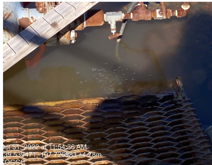
Well head leaking
