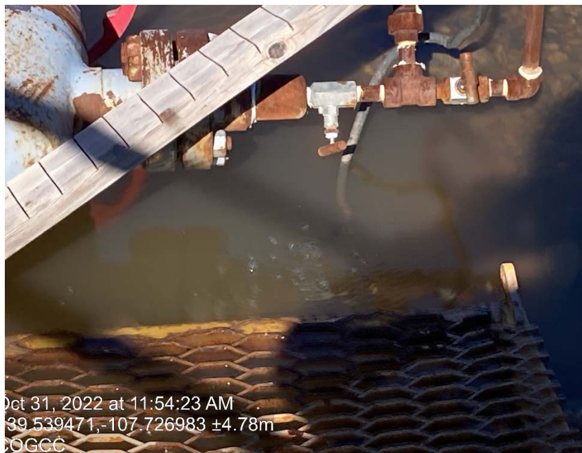
Well head leaking
