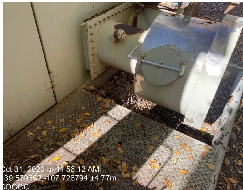
Debris under lit burner
