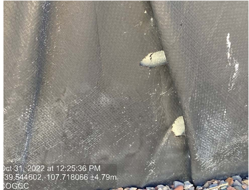
Holes in containment
