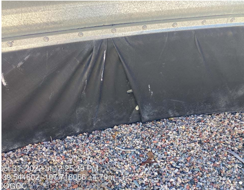
Holes in containment
