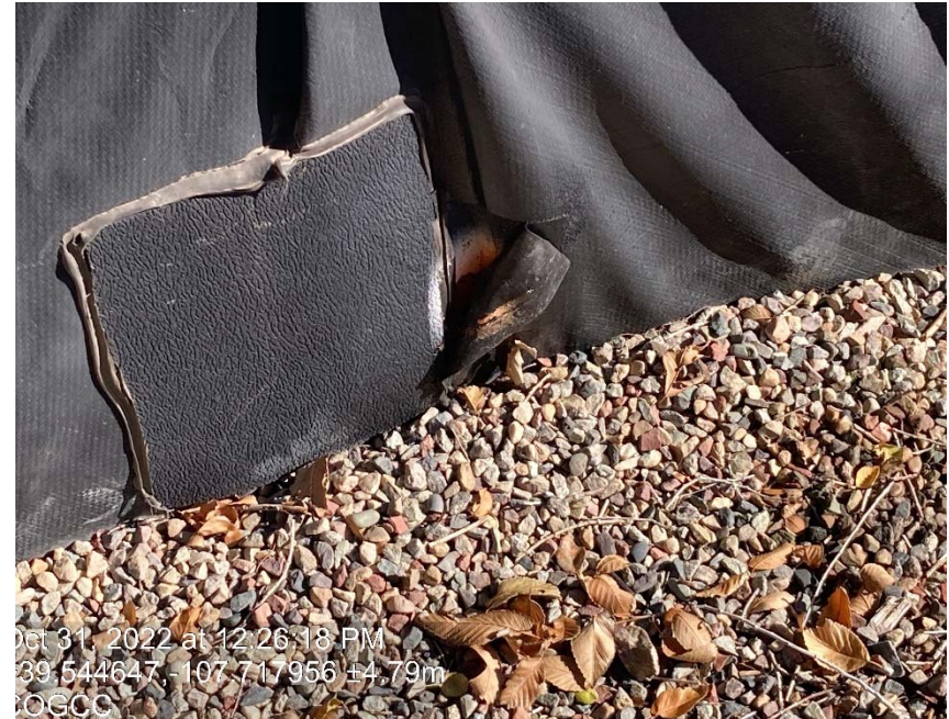
Holes in containment
