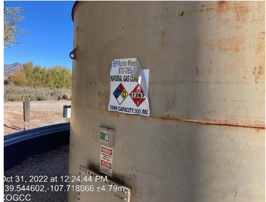
Labeling falling off
