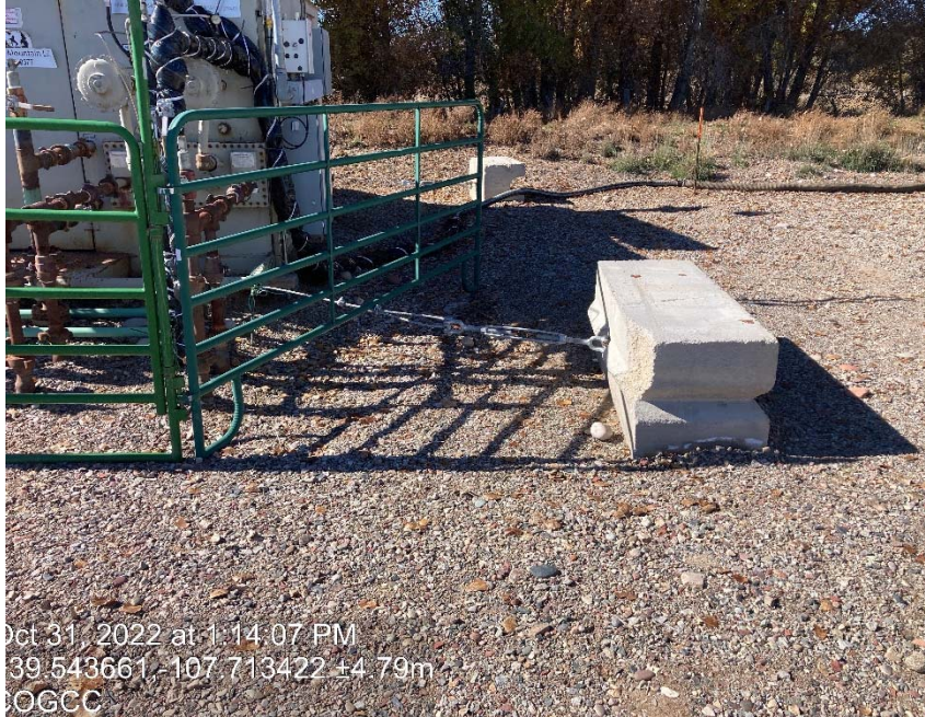
Separator anchored
