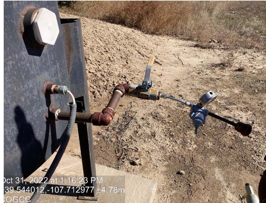
Stored equipment disconnected from all piping
