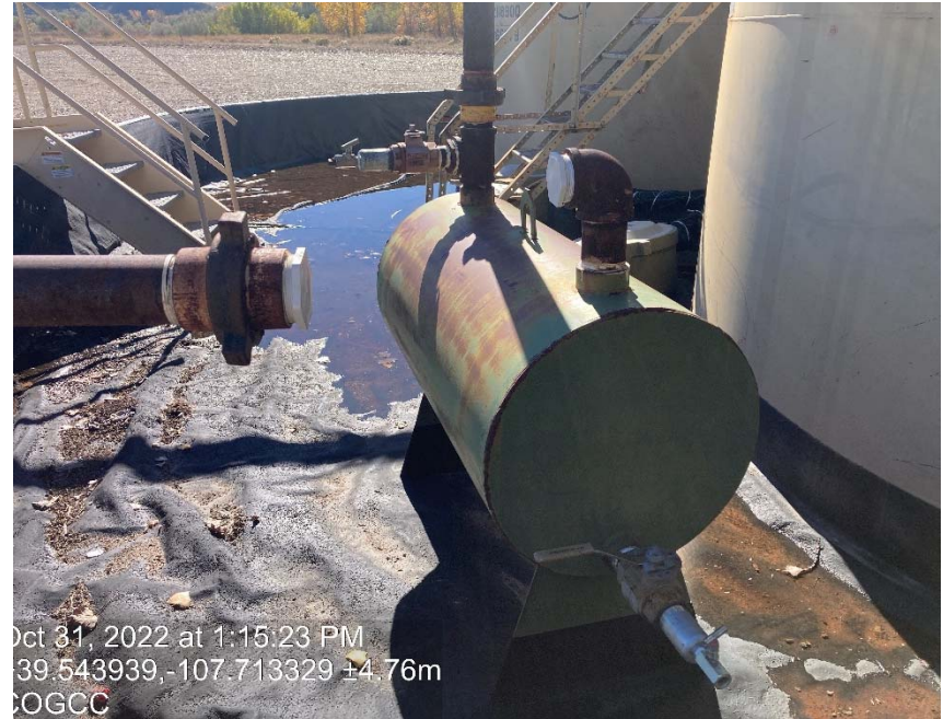
Piping from tanks to stored equipment is disconnected
