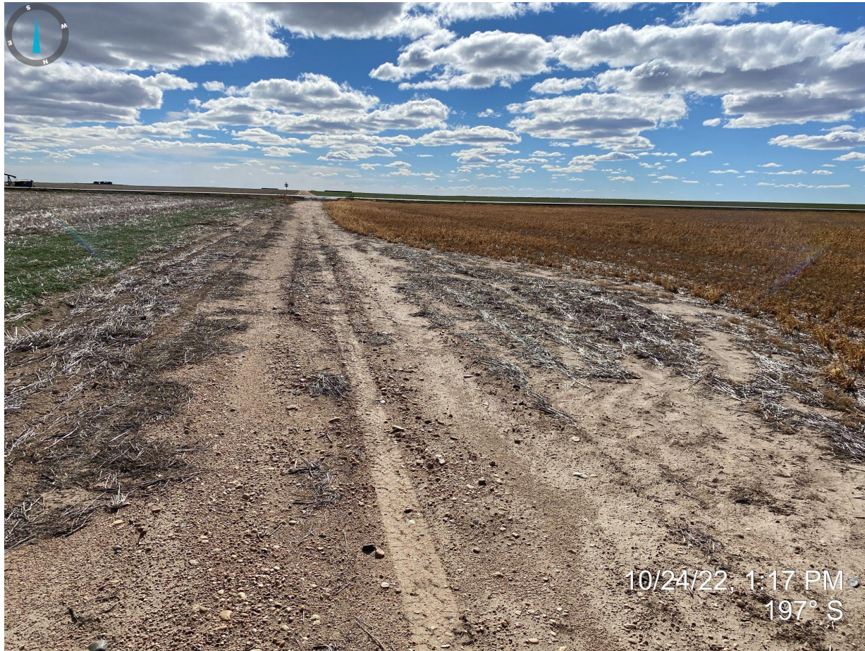
Photo 1. Taken from access road, facing south. Photo illustrates the access road has not been reclaimed with presence of road base/gravel.
