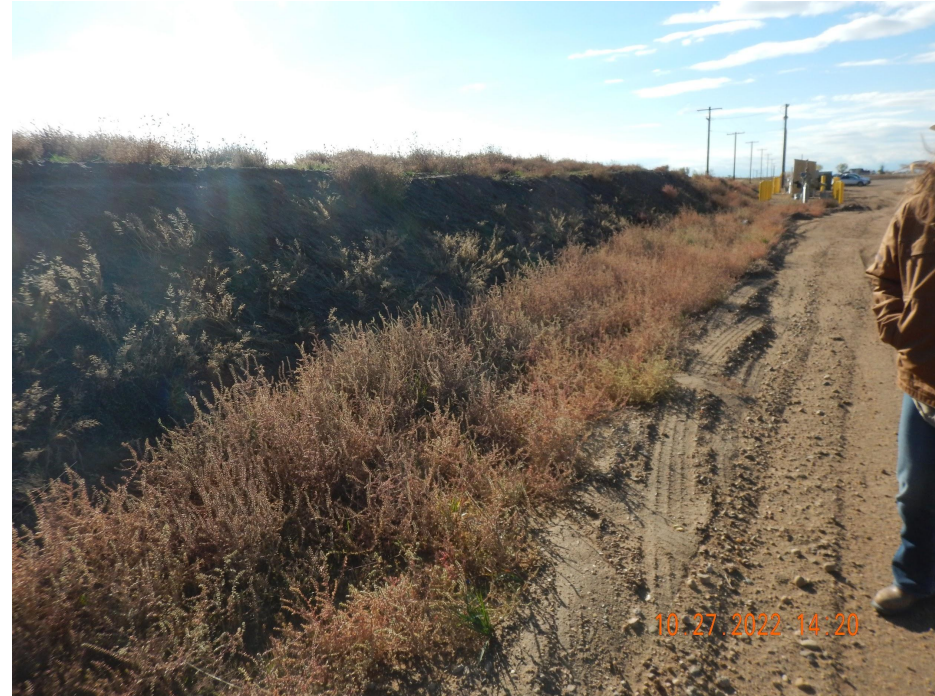
Photo 14. Photo taken southeastern location, facing West. Photo illustrates a cut slope needing weed maintenance and stabilization.
