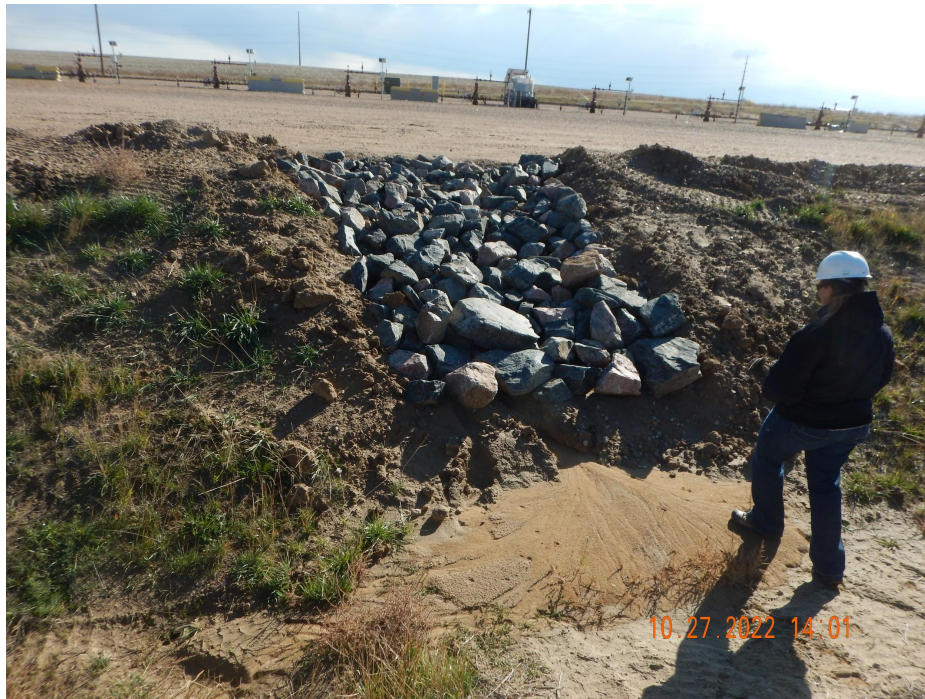
Photo 9. Photo taken from the northern stormwater BMP area, facing South. Photo illustrates erosion undercutting the riprap because there is no liner.
