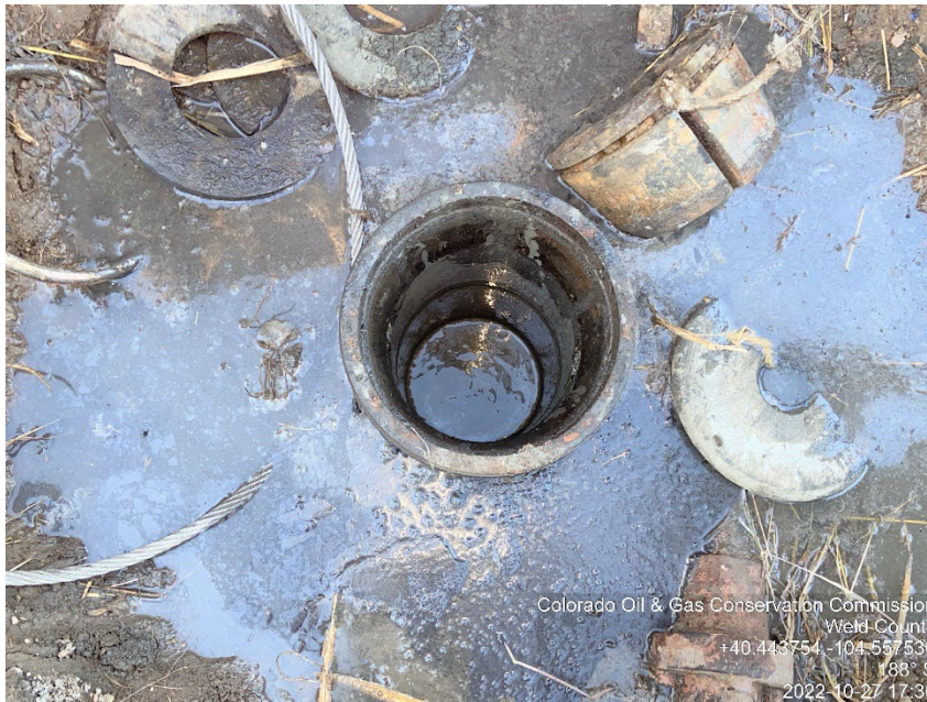
Photo #3 Noffsinger 22-33 Wellsite Plugged & Abandoned | PA Plugging Operations: Cementing | WK Cement to surface
