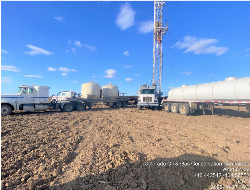
Photo #1 Noffsinger 22-33 (05-123-20237) Wellsite Plugged & Abandoned | PA Plugging Operations: Cementing | WK Final plugs / Cement to surface
