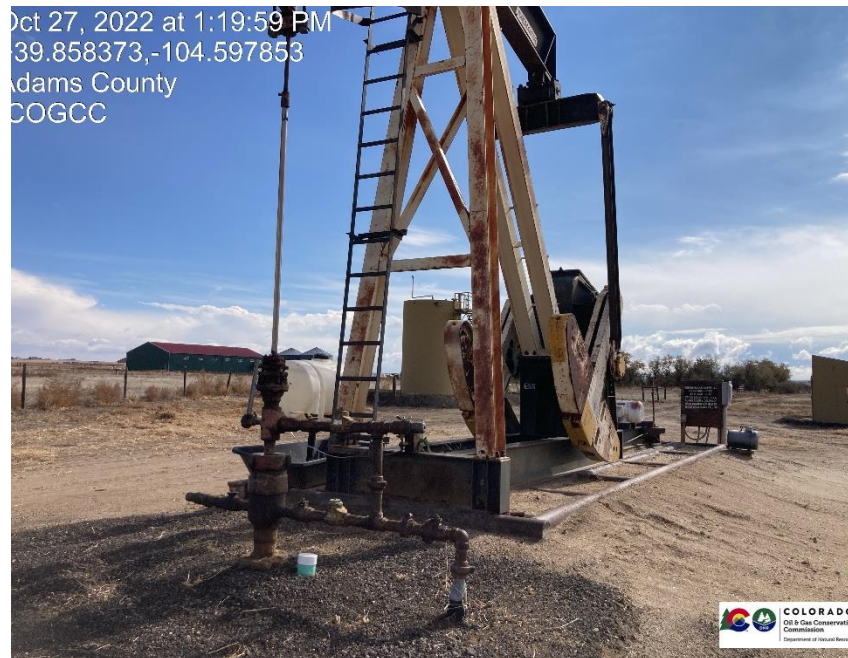
Pic 2 wellhead / pump jack
