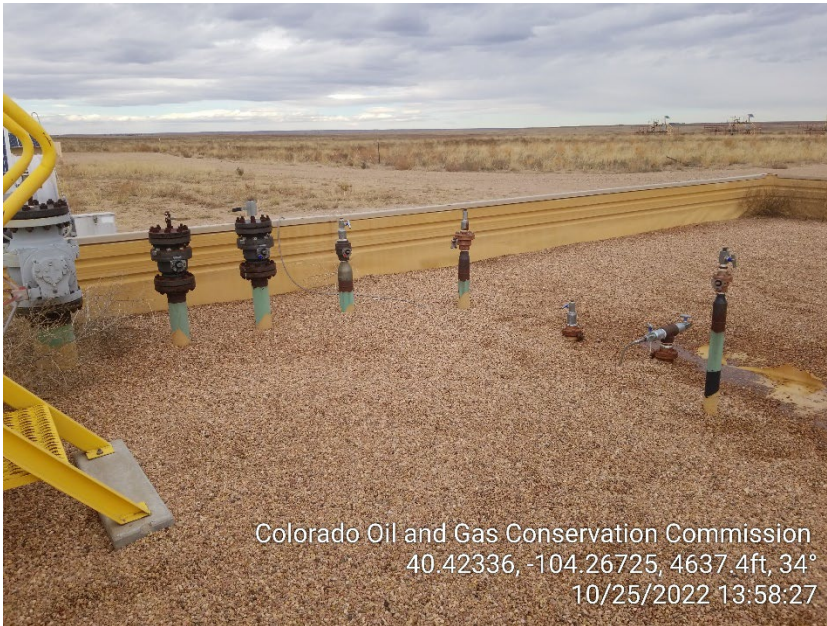
Photo 5 – Unmarked Riser at Separators
