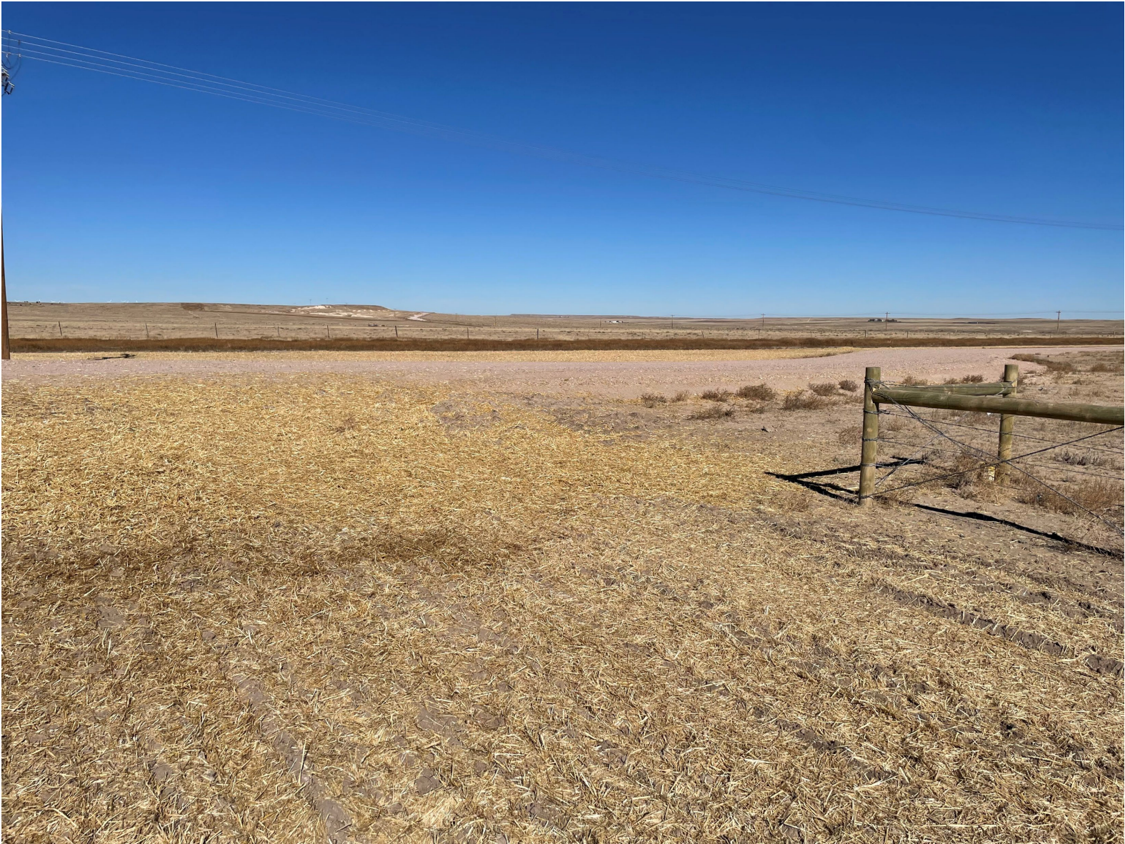
Interim reclamation has commenced. Pad has been pulled back and seeding with straw mulching has been completed. Standing near entrance, looking north.
