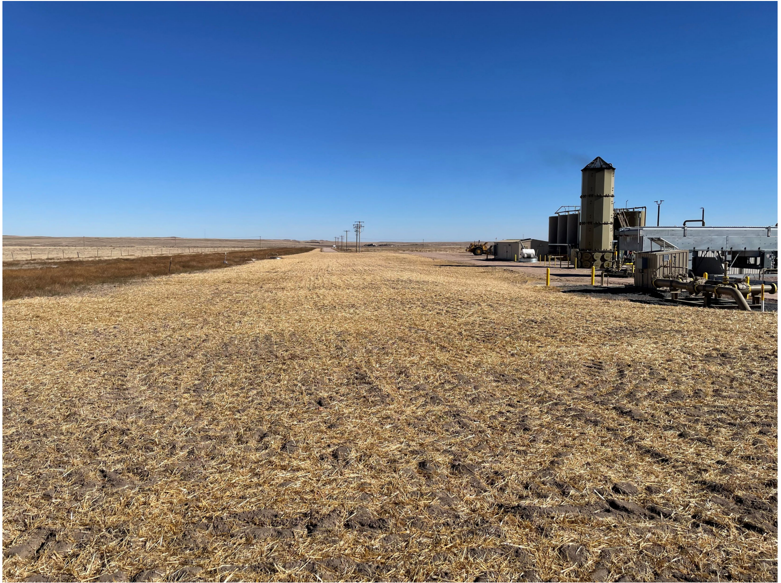
Interim reclamation has commenced. Pad has been pulled back and seeding with straw mulching has been completed. Standing near northwest corner, looking east.
